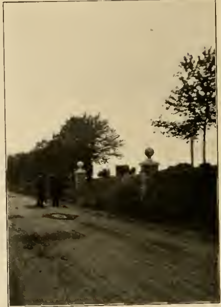
Main Entrance to Creighton Manor
