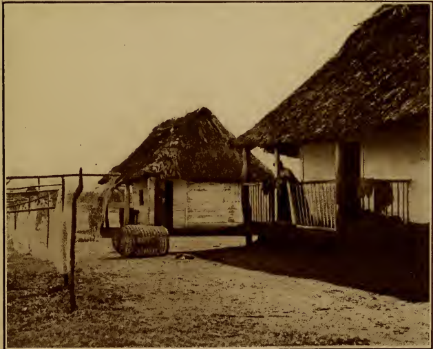
CUBAN VILLAGE HOUSE UNDER CONSTRUCTION. FISHERMEN'S HOMES, ESPERANZA, CUBA.
