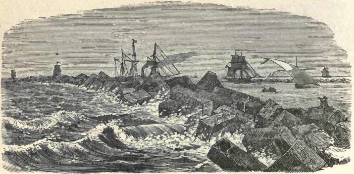
FIG. 123.— One of the Breakwaters at Port Saïd.
