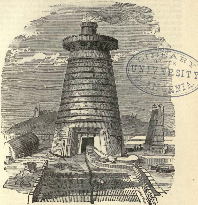
FIG. 17.— Blast Furnace.
