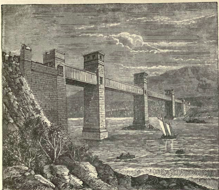
FIG. 138.— Britannia Bridge, Menai Straits.
