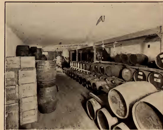
STOREROOM FOR BULK GOODS. 4th Floor, Nos. 24 and 26 North 9th Street.
