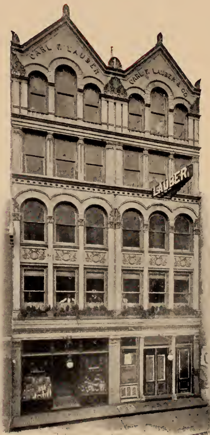
Nos. 24 and 26 N. 9th Street.
