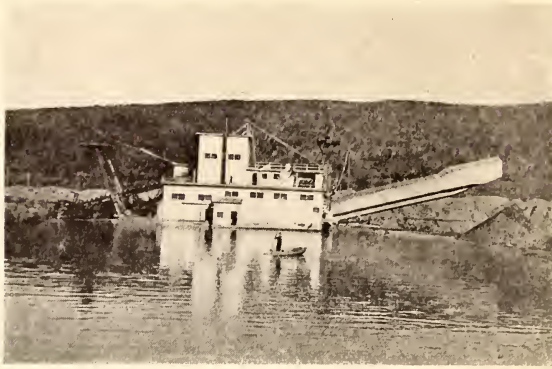
Dredge used in the large-scale placer mining of Interior Alaska.
