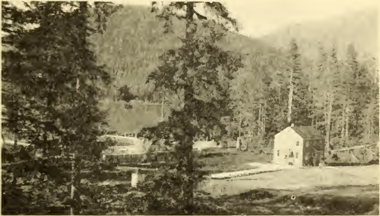
General view of Petersburg Sub-Station No. 2.
