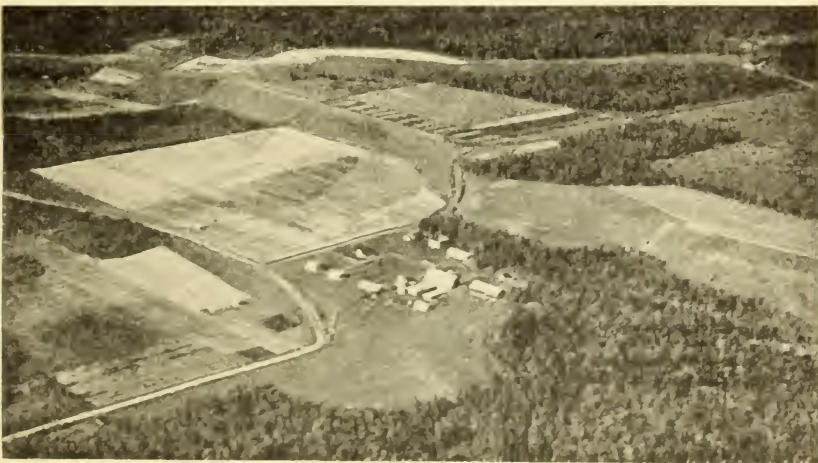
The Matanuska Sub-Station No. 1 from the air. The benchland topography and relatively heavy forest growth are well shown in this photograph.
