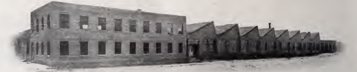
The skylights all face north. The roof is of saw-toothed variety. There are no dark corners in this factory and the finest scale can be read anywhere under ordinary daylight.
