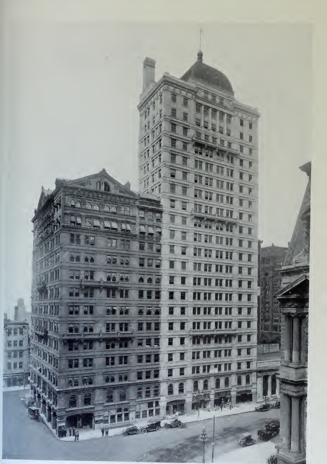
COMMERCIAL TRUST BUILDING, PHILADELPHIA
