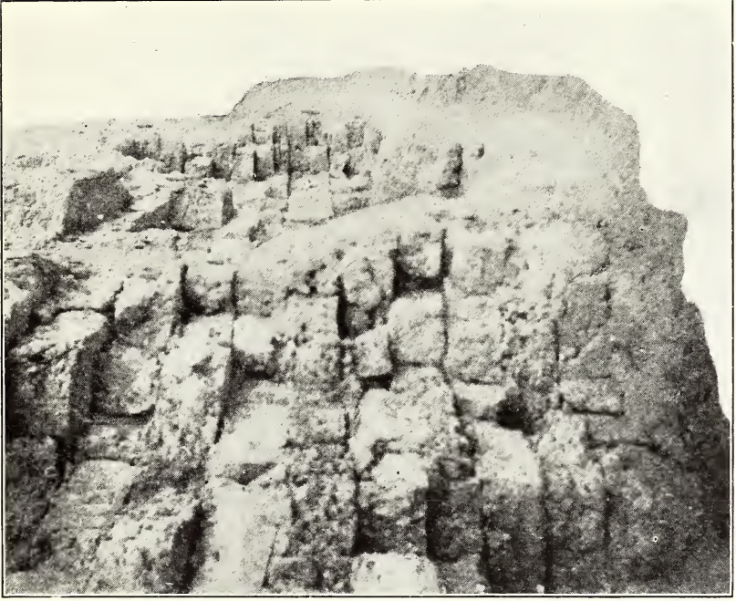
CRUMBLING WALLS OF REI
