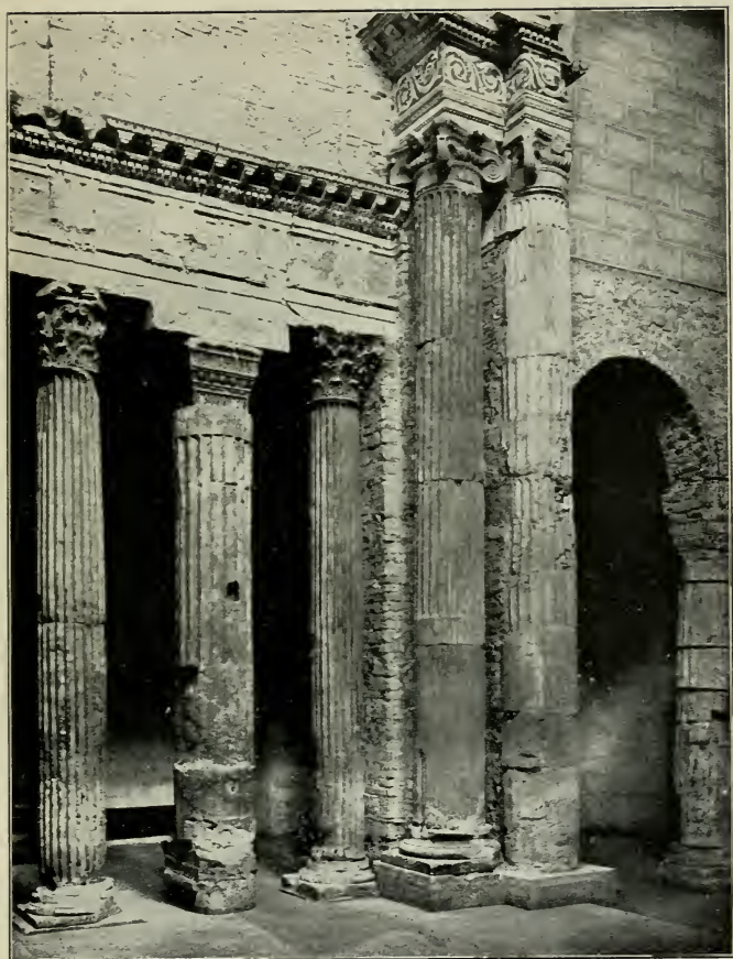
Spoletto, Interior of the Church of the Crocifisso showing profuse and confused use of Roman material
