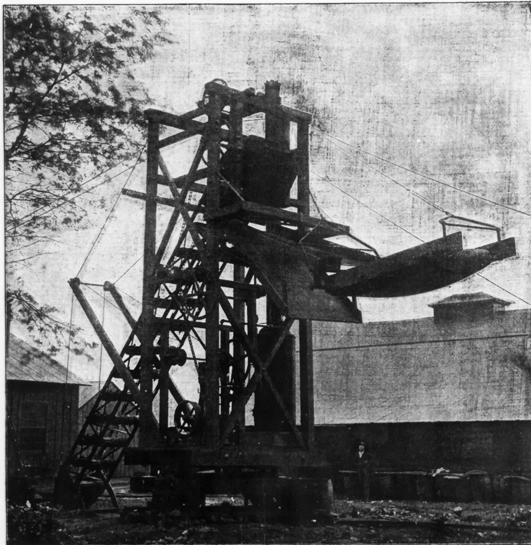
THE JEFFREY PORTABLE ELEVATOR, SCREEN AND CONVEYOR.
