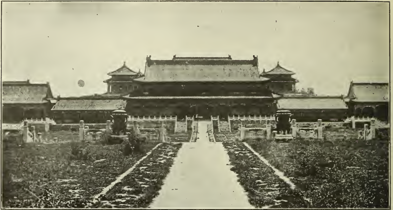
A STYLE OF ARCHITECTURE WHICH IS RAPIDLY DISAPPEARING IN SOME PARTS OF CHINA
