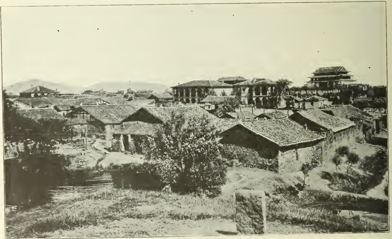
THE MISSION BUILDINGS AT NANCHANG.
