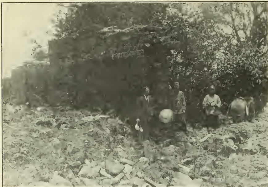
A MOUNTAIN-TOP RUIN OF AN OLD CASTLE OF A FORMER NOSU CHIEFTAIN IN YUNNAN. STANDING BY THE WALL ARE MR. PARKER AND MR. GOBY, THE LATTER NEAREST THE CENTRE OF THE PICTURE. THE NATIVE IS OF THE LISU TRIBE
