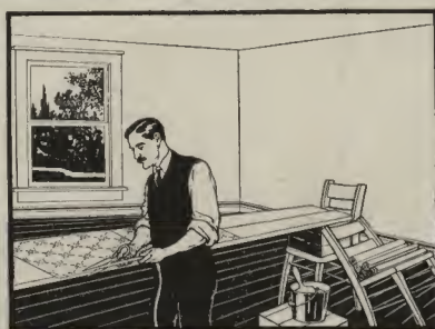
ILLUSTRATION No. 2. Trimming a strip of wall paper after it has been pasted.
