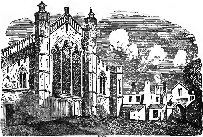
WEST END OF SAINT GEORGE'S CHAPEL
