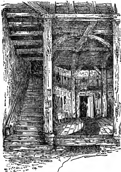
INTERIOR OF THE CURFEW TOWER
