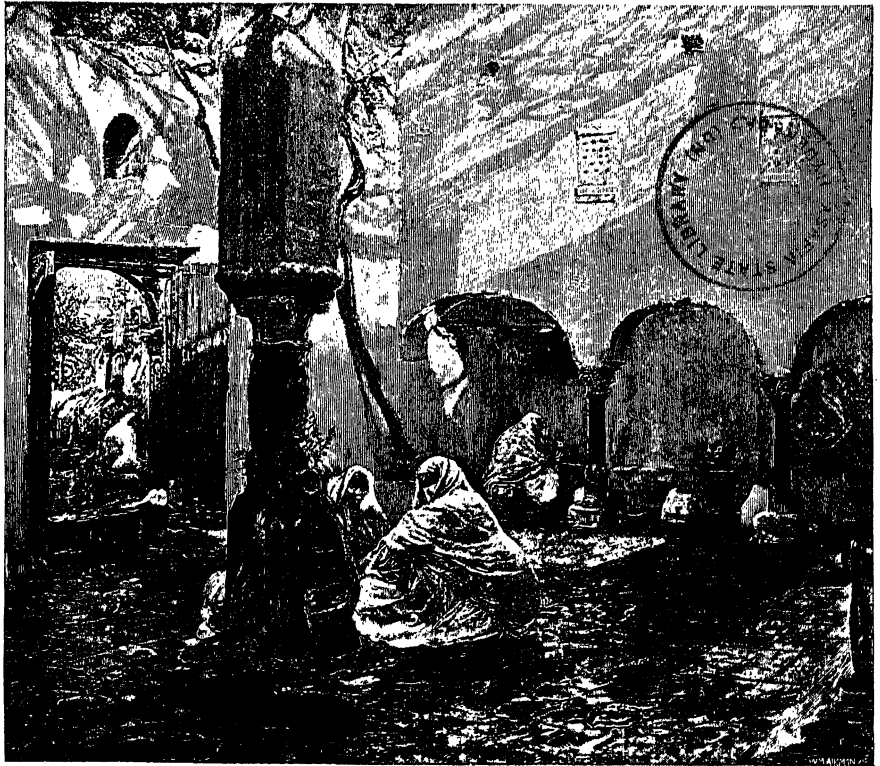
COURT OF THE KHOUBA AT BELCOUR.
