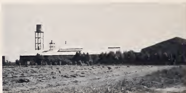
Right. Drainage water from the Gomez Palacio plant is used to irrigate surrounding alfalfa fields.
