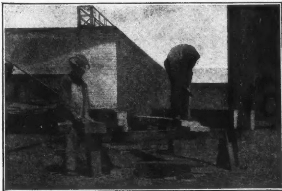
Timber must be seasoned air-dry, and completely framed—all bolt holes drilled, tenons and mortises cut—before treatment.
