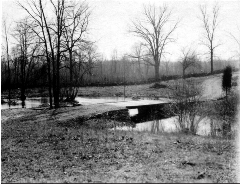
Figure 2.79. The new bridge built in 1924 and recently cleared overgrown pastures at the future site of Val-Kill looking southwest from near the future site of Stone Cottage, ca. 1925. This is the same view as in the previous figure. (Photograph 48: 224039[6], Franklin D. Roosevelt Library.)
