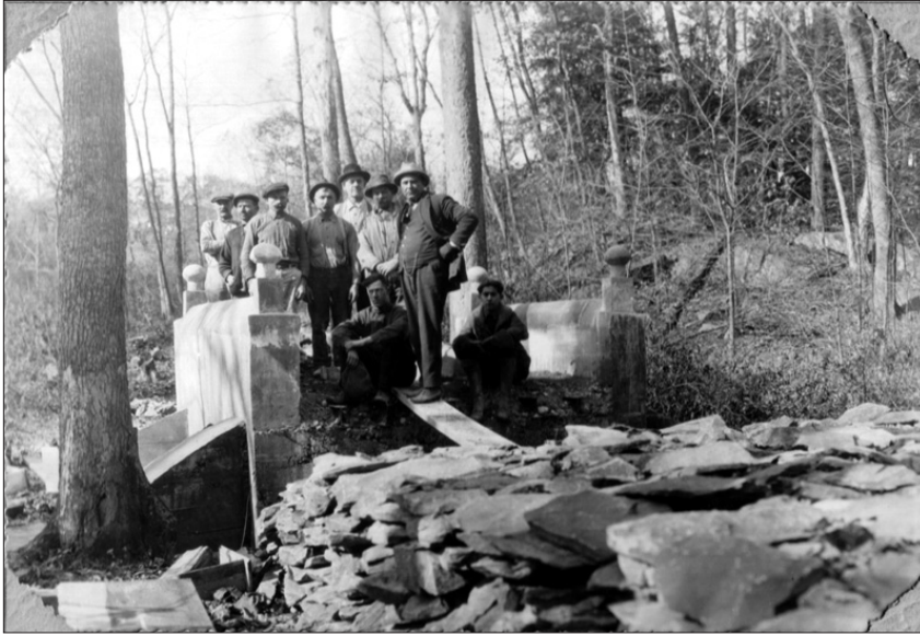
Figure 2.68. Looking west at the new concrete bridge carrying Farm Road over the Maritje Kill nearing completion, October 1923. In the foreground is the rubble-fill causeway approach. (Photograph NPx 48-22-3837[5], Franklin D. Roosevelt Library.)
