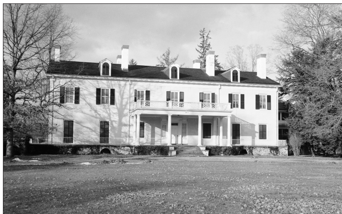
Figure 2.34. Bellefield house as redesigned in 1909 in a Colonial Revival style, view looking west, ca. 1950. The original house corresponds with the center three bays. (Photograph R2162, Roosevelt-Vanderbilt National Historic Sites.)
