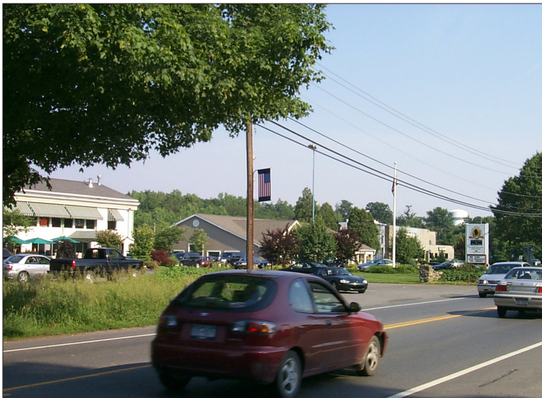
Figure 2.177. Commercial development on the Home Farm looking southeast from the library entrance drive, 2003. The middle building was constructed after 1970; the others date to the late 1940s and early 1950s. The water tower in the distance is near Saint Andrews Road, outside of the estate. (SUNY ESF)
