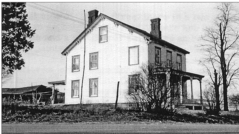
Figure 2.143. The Rohan farmhouse, looking northwest from the intersection of Cream Street and Dutchess Hill Road, 1945. ("Appraisal of the Franklin D. Roosevelt Real Estate," April 12, 1945, O'Connor and Farber Papers, Franklin D. Roosevelt Library.)
