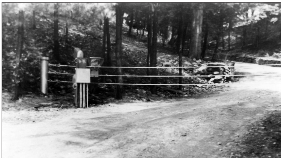
Figure 2.96. Typical wartime crash barrier and electric eye, looking south along the road to the Duplex on the Wheeler Place with the stone wall-lined River Road in the background, ca. 1942. (Photograph Px 80-26 [2], Franklin D. Roosevelt Library.)
