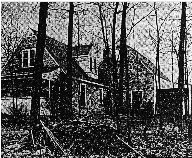
Figure 2.172. Looking southeast at Top Cottage during Elliott Roosevelt's ownership showing addition of dormer, windows, and porch on north wing (left), loss of trees surrounding the house, and unkempt conditions, ca. 1952. Compare with the ca. 1940 photograph of Top Cottage in figure 2.146. ("Roosevelts Sell 500-Acre Tract at Hyde Park," New York Herald Tribune , April 18, 1952.)
