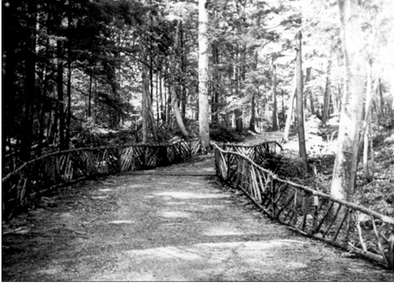
Figure 2.24. Looking northeast along River Road in the lower woods of the Boreel Place showing the rustic bridge and railings built in ca. 1870 across the unnamed creek, photographed ca. 1898. (Photograph NPx 49-8:23, Franklin D. Roosevelt Library.)
