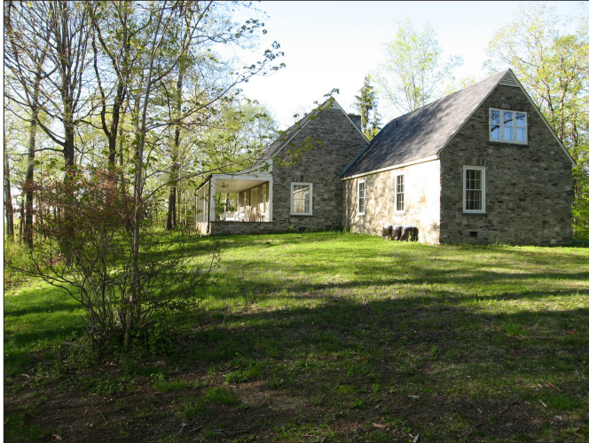
Figure 2.184. Top Cottage looking north following its restoration completed in 2001, photographed 2007. (SUNY ESF.)
