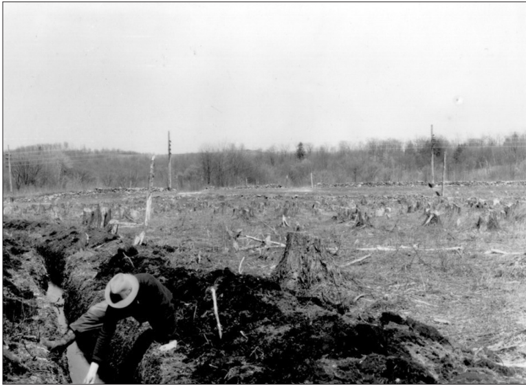
1.13. The cleared and drained Tamarack Swamp on the Roosevelt Estate (Tompkins Farm) prior to replanting, looking east toward Creek Road, April 1933. The person inspecting the ditch may be Nelson Brown. (Photograph 48-224000(3), Franklin D. Roosevelt Library.)
