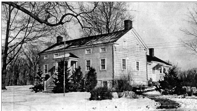
Figure 2.133. The Hughson farmhouse looking northeast from the entry road (Pell's Lane), 1945. At the time of the photograph, the house was known as the Linaka Cottage. ("Appraisal of the Franklin D. Roosevelt Real Estate," April 12, 1945, O'Connor and Farber Papers, Franklin D. Roosevelt Library.)
