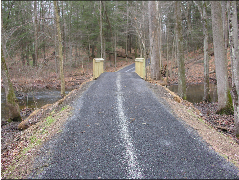
Figure 2.178. Looking west along Farm Road on the Home Farm, rebuilt in 2008 as Roosevelt Farm Lane linking Val-Kill with the FDR Home and Library. The bridge spans the Maritje Kill over the remains of a concrete arched bridge built in 1923 (see fig. 2.68). (National Park Service.)
