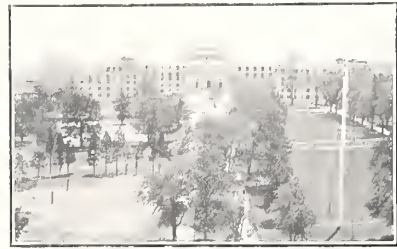
VIEW FROM THE ACADEMIC BUILDING.
