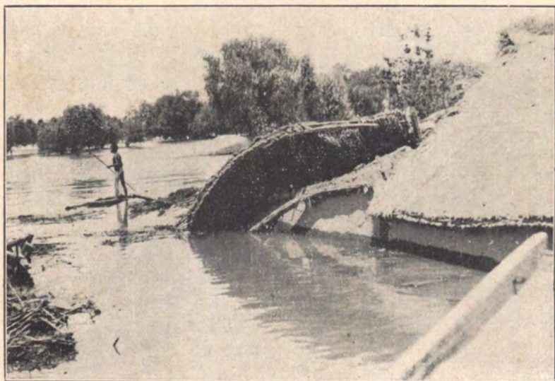
屋宇冲倒 Houses collapsed
