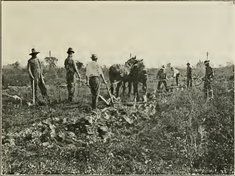
Stripping the surface loam off a clay field.
