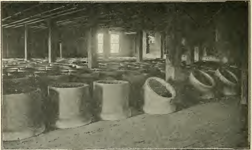
Twenty-four-inch pipe on drying floor, Mimico, Ont.
