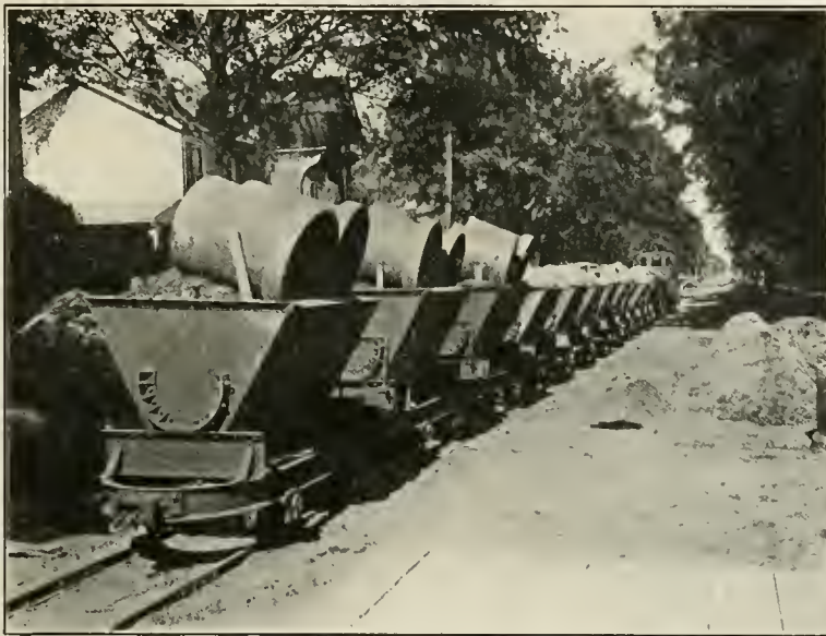
Sewer pipe used on the Good Road construction, Toronto-to-Hamilton Highway.
