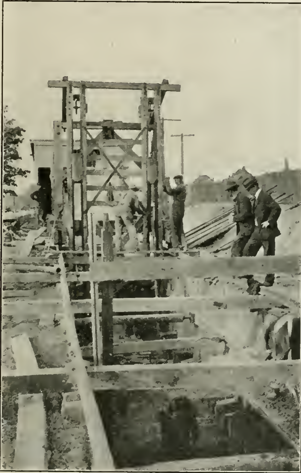
Laying a 33" dia. sewer in quicksand, Peterboro', Ont.
