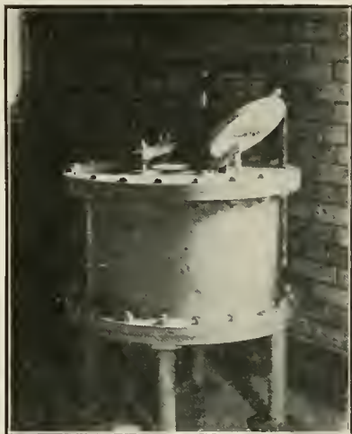
Apparatus at Lindsay for elevating alum or a solution to storage tanks.
