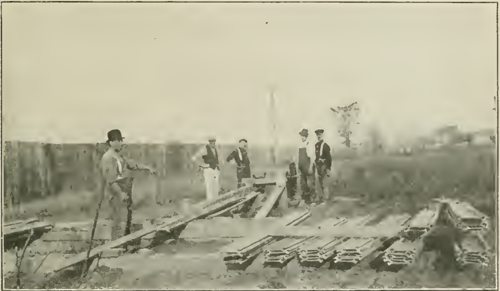
Straightening the steel sheeting, Peterboro', Ont.
