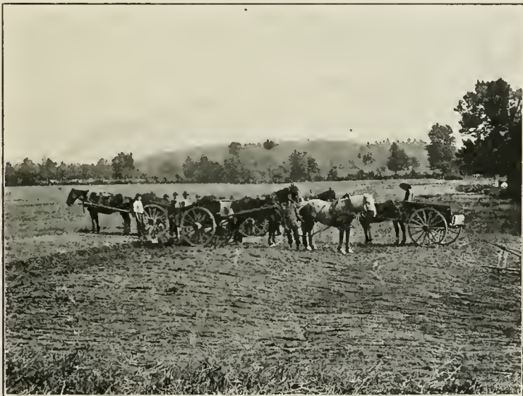
Stripping sewer-pipe clay near Hamilton, Ont.
