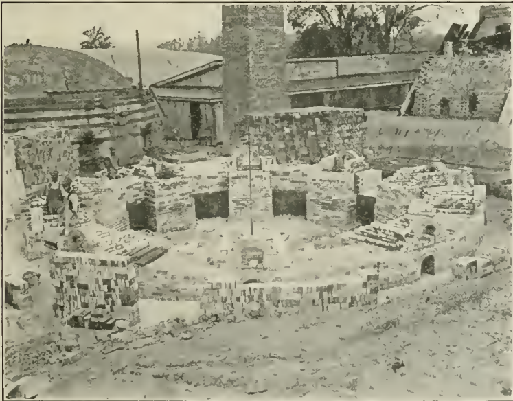
Brick kiln under construction, Rymal, Ont.
