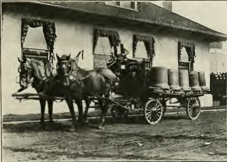
Office and dray, Hamilton-Toronto Sewer Pipe Co., Ltd.
