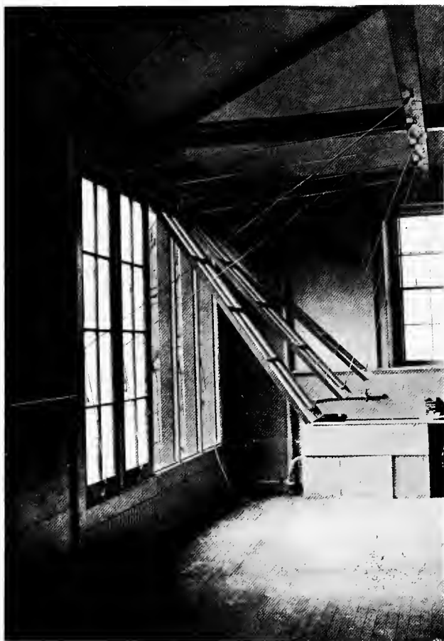
The windows in the Providence school are hinged at the top and can be raised against the ceiling by cords and pulleys
