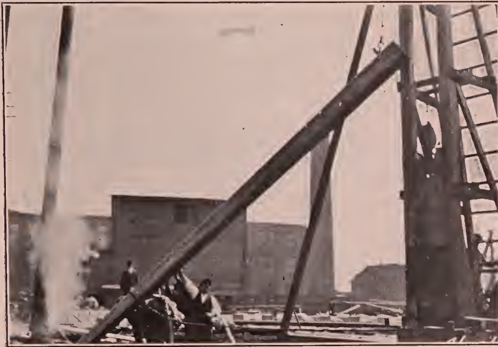
Fig. 40—Hoisting Concrete Pile Into Driving Position.
