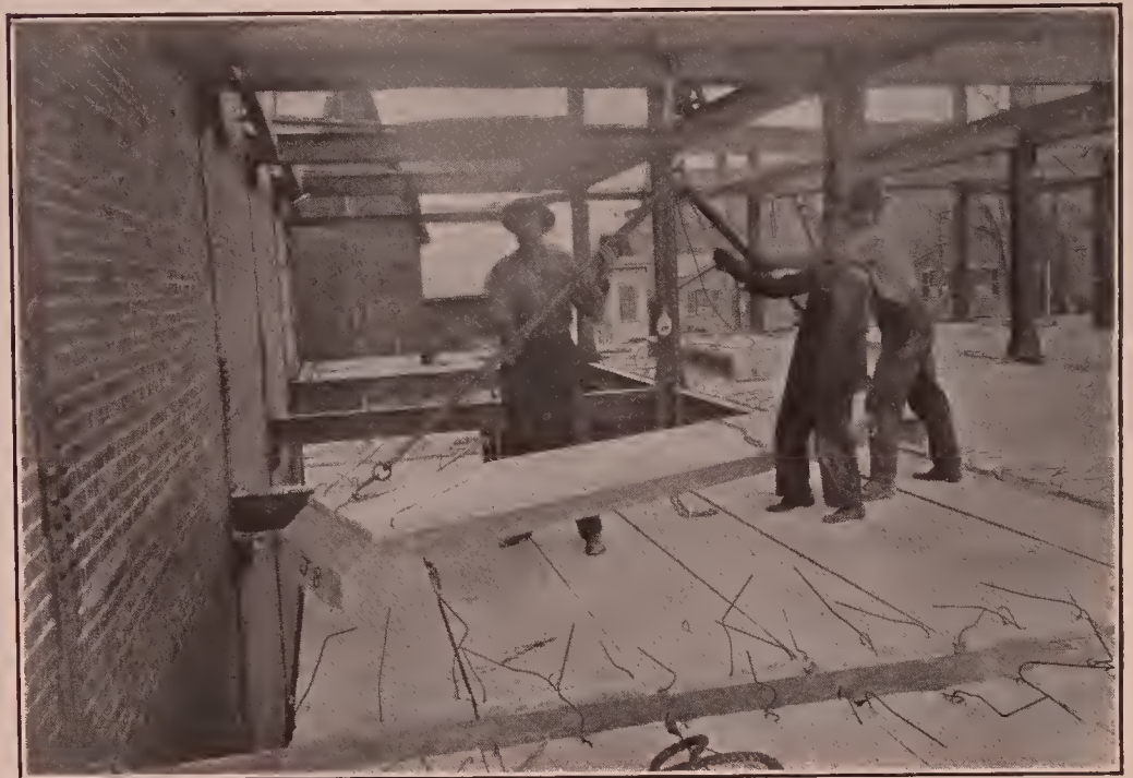
Fig. 55—Method of Handling Separately Moulded Floor Section.
