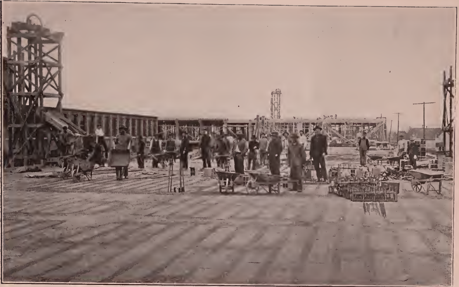
Fig. 51—Concrete and Tile Floor Under Construction.
