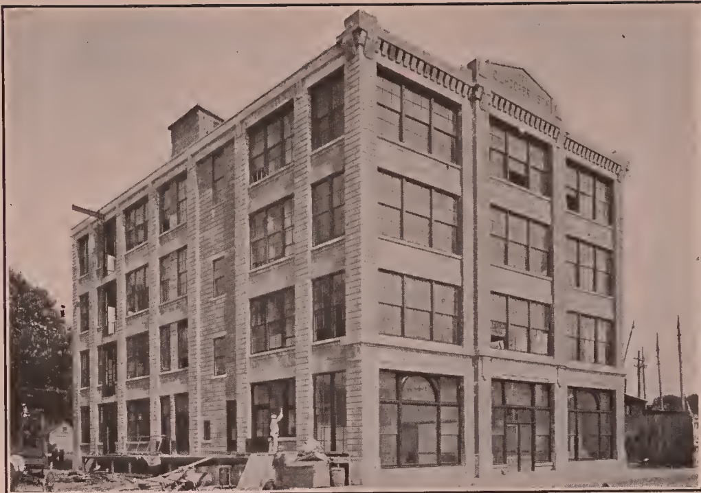
Fig. 93—Concrete Block Walls, Salem Laundry.
