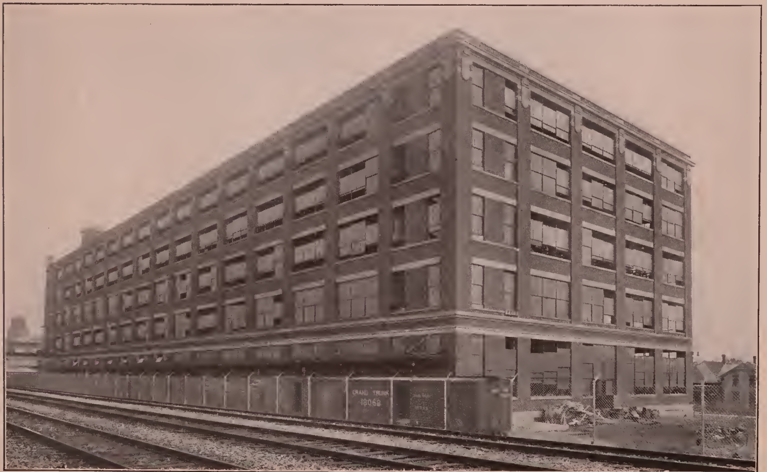
Figure 106—General Electric Company Building No. 26, Fort Wayne, Ind. Harris & Richards, Architects. Wells Bros., Contractors
