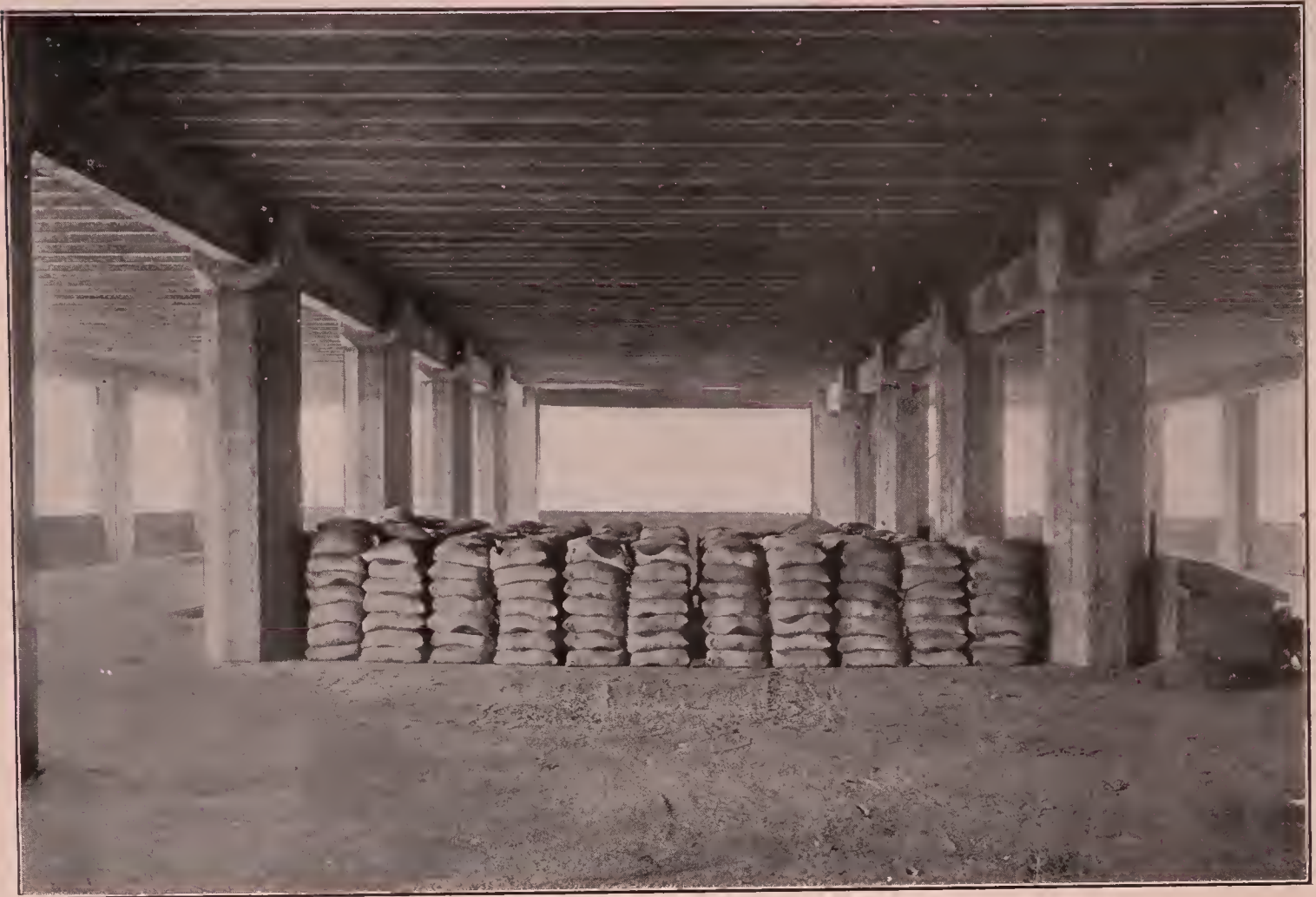
Fig. 46—View of Interior of Bush Model Factory No. 2
