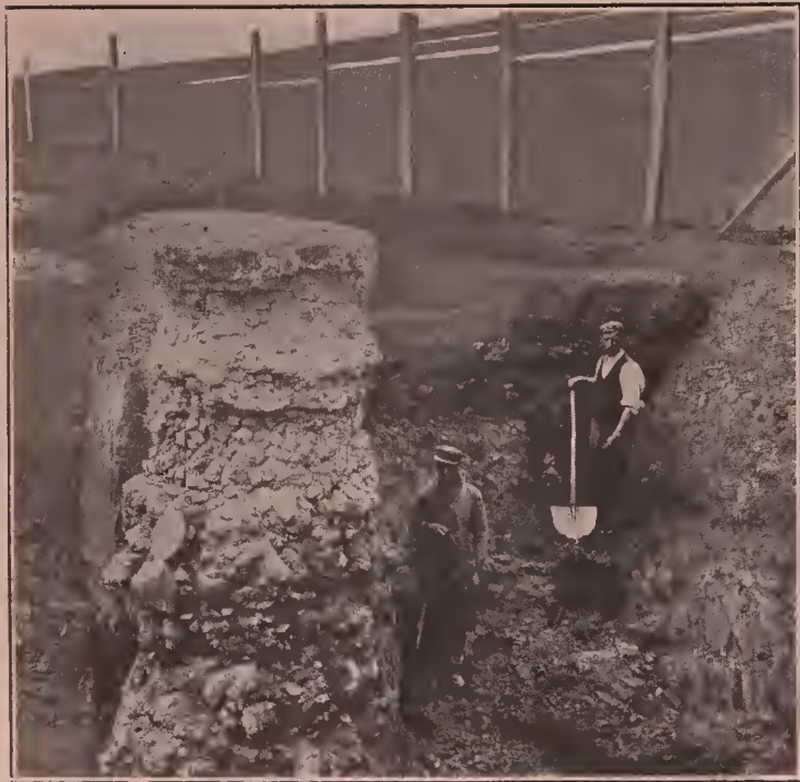
Fig. 101—Hennebique Compressed Pile—See page 88.
