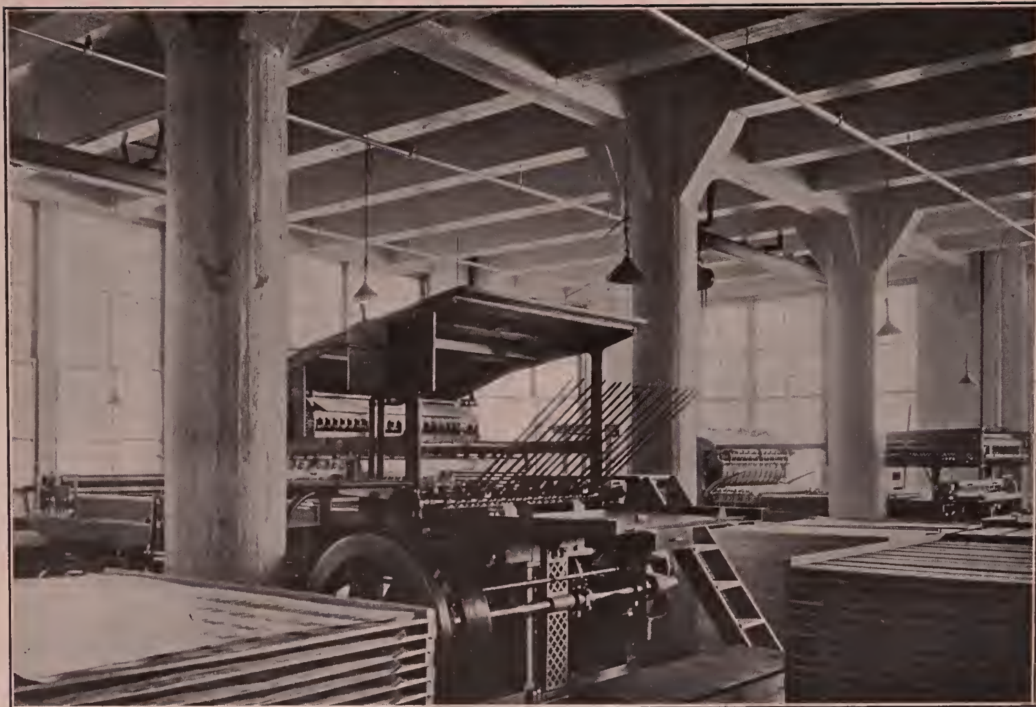
Fig. 13—Interior of Ketterlinus Building, Showing 20-Ton Lithographic Press.
