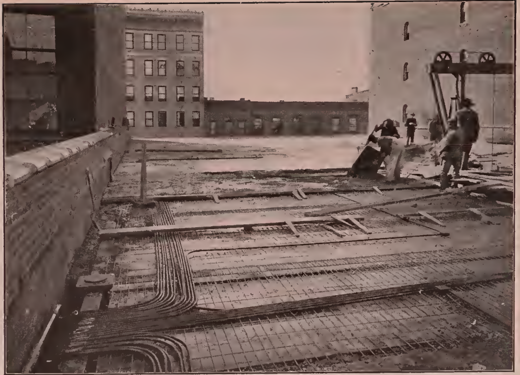
Fig. 86—Laying Clinton Welded Wire in Decauville Garage, New York.
