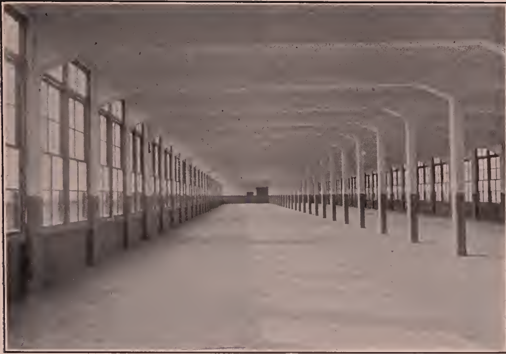
Fig. 39—Interior View of Hose Building.
