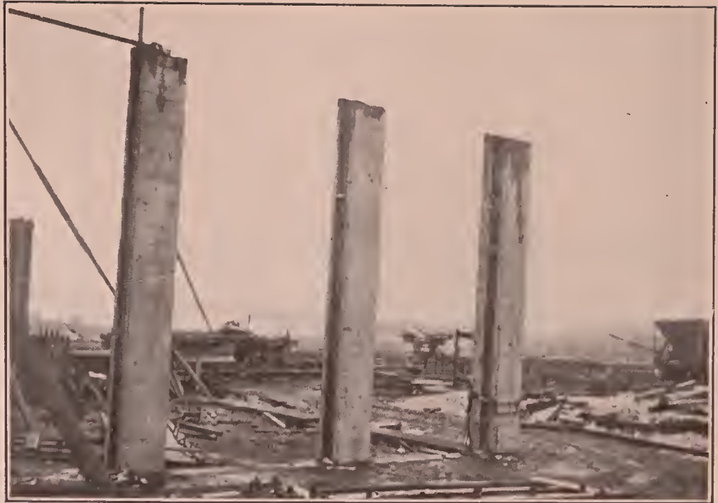
Fig. 60—Wall Piers for The Atlas Portland Cement Company Building.
