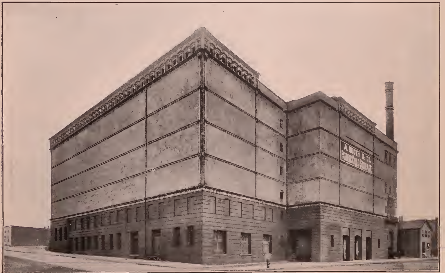
Fig. 108—A. Booth & Company, Detroit, Mich. John Scott & Company, Architects. Concrete Steel & Tile Construction Company, Contractors
