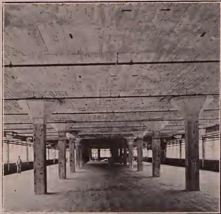
Fig. 26—Interior of Loading Building, Winchester Repeating Arms Company
