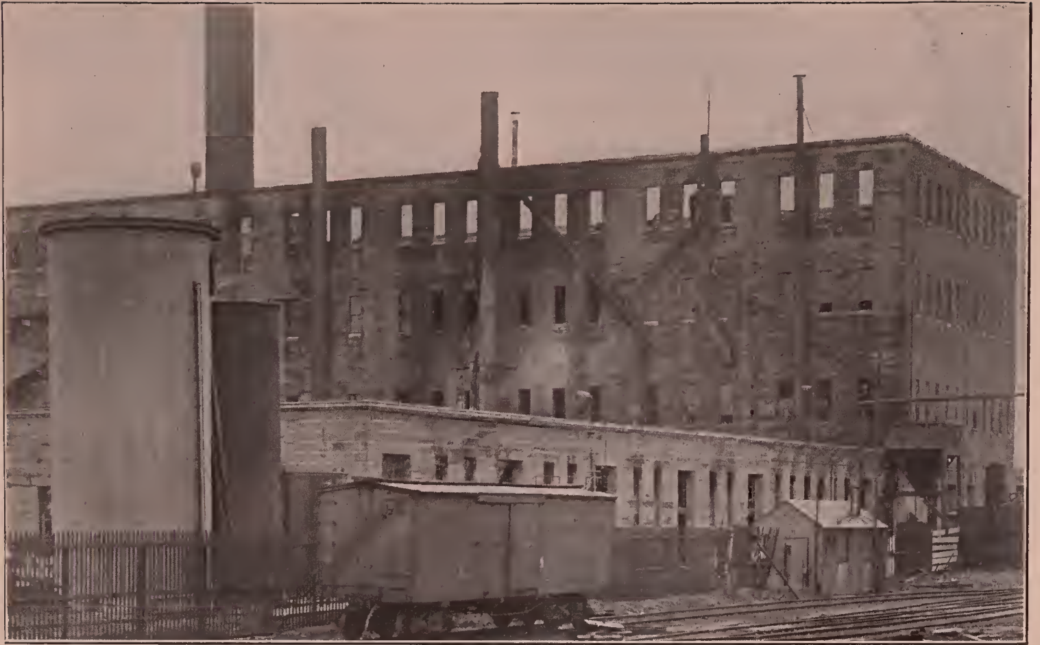
Fig. 76—View of Refinery After the Fire.
