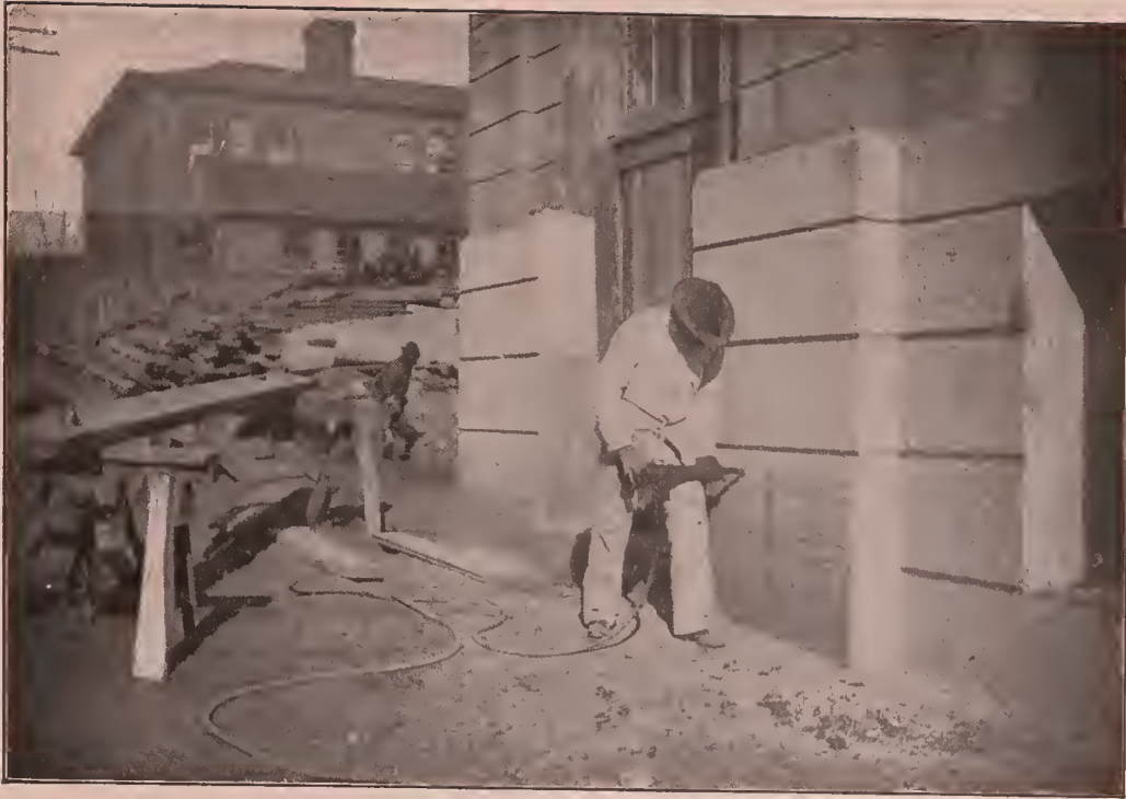
Fig. 95—Tooling the Surface of Friedenwald Building Walls.
