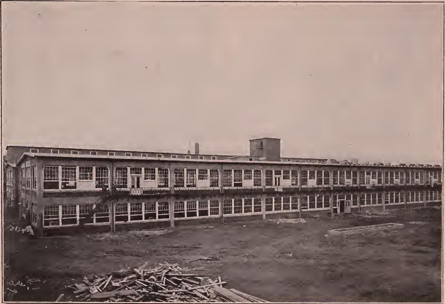
Fig. 23—Loading Buildings, Winchester Repeating Arms Company.
