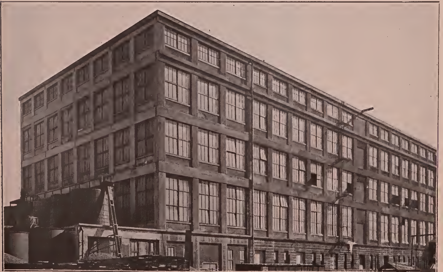
Fig. 77—View of Refinery, Including New and Old Structures.
