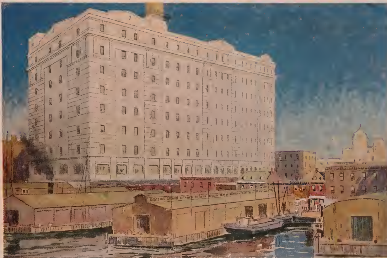
Reinforced Concrete Terminal Warehouse—Baltimore and Ohio Railroad, New York M. A. Long, Engineer Turner Construction Company, Contractors
