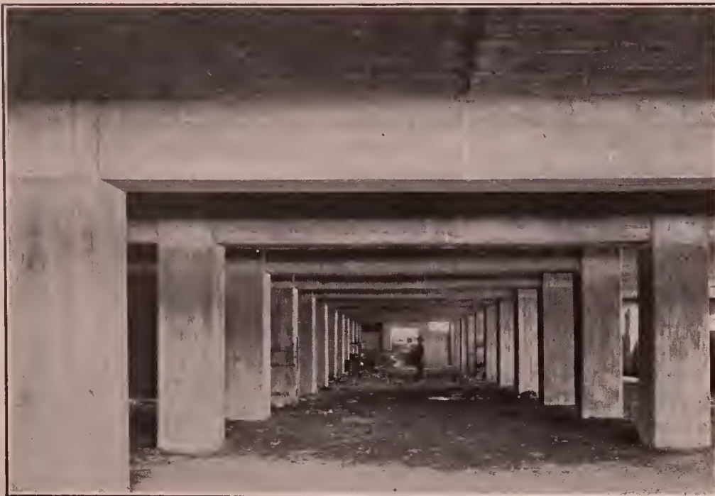
Fig. 6.—Interior of Basement, Carter's Ink Factory.
