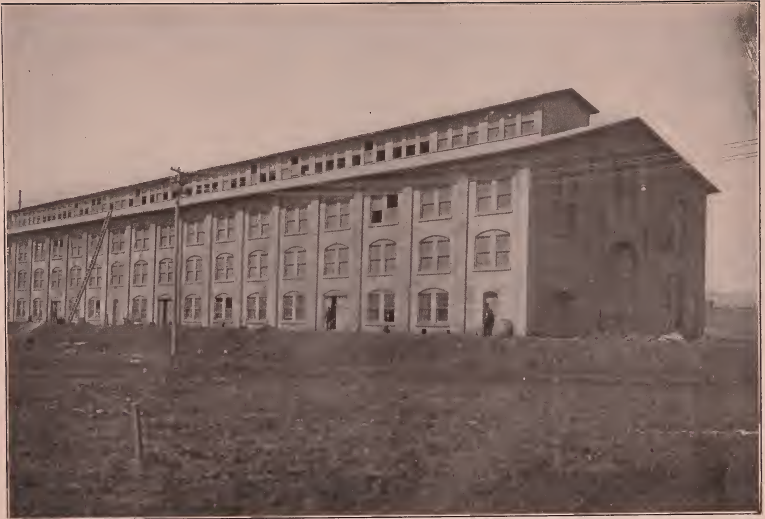
Fig. 57—Blacksmith and Boiler Shop of The Atlas Portland Cement Co. at Northampton, Pa.
