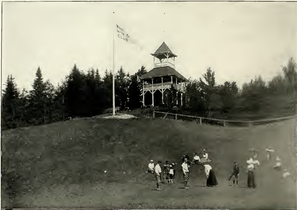
OBSERVATORY AND FIRST TEE—TWIN MOUNTAIN HOUSE LINKS.
