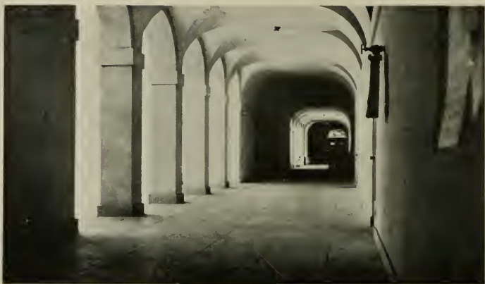
CORRIDOR, GARFIELD SCHOOL BUILDING, BERKELEY Coxhead & Coxhead, Architects W. H. Ratcliff, Jr., Supervising Architect
