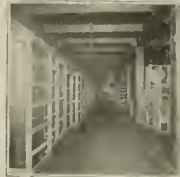
Storage Tanks, San Francisco Warehouse
