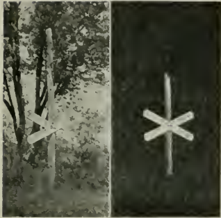
Day and night views of a railroad crossing sign. A special holder is fitted to a street series socket which carries a glass reflector bright red on the outside and white opal on the inside. A sixty candle-power street series lamp is used.
