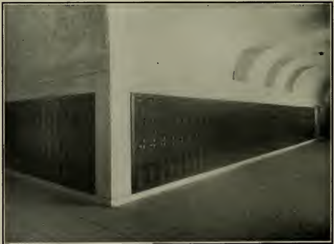
DURAND STEEL LOCKER INSTALLATION IN GARFIELD SCHOOL BUILDING, BERKELEY
