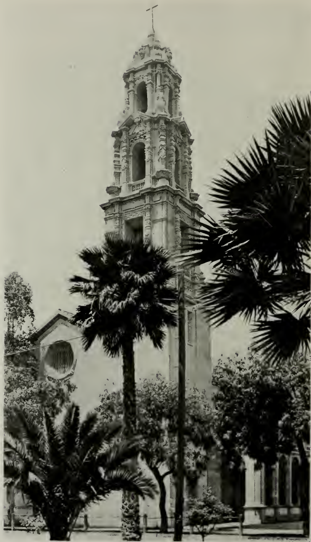
FIRST CONGREGATIONAL CHURCH, RIVERSIDE MYRON HUNT, ARCHITECT
