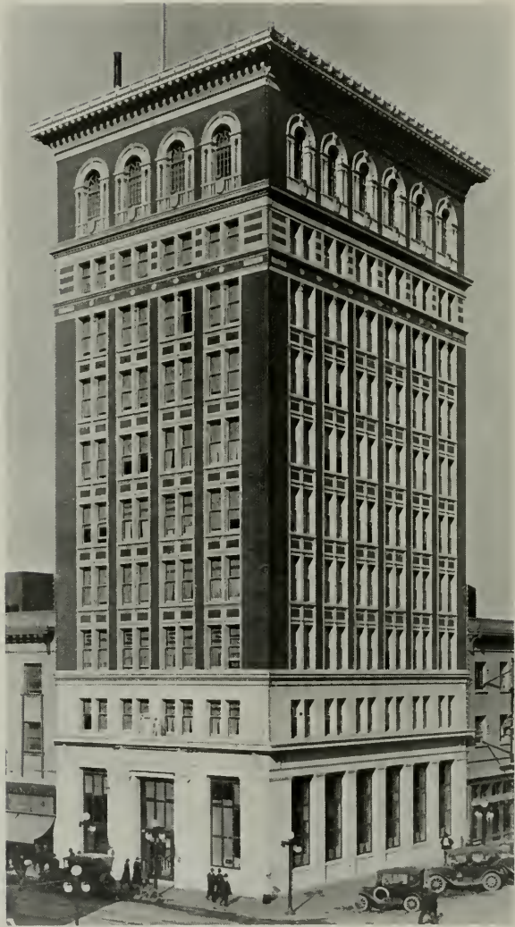
COMMERCIAL AND SAVINGS BANK BUILDING, STOCKTON, CALIFORNIA L. B. DUTTON, ARCHITECT STONE & WRIGHT, ASSOCIATES
