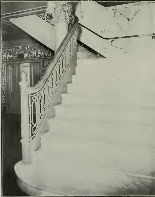
MARBLE AND BRONZE STAIRCASE, ORPHEUM THEATER, LOS ANGELES G. ALBERT LANSEBURGH ARCHITECT
