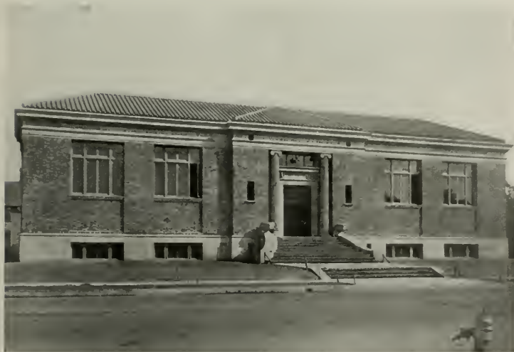
VERNON BRANCH LIBRARY Kysor & Biggar, Architects
