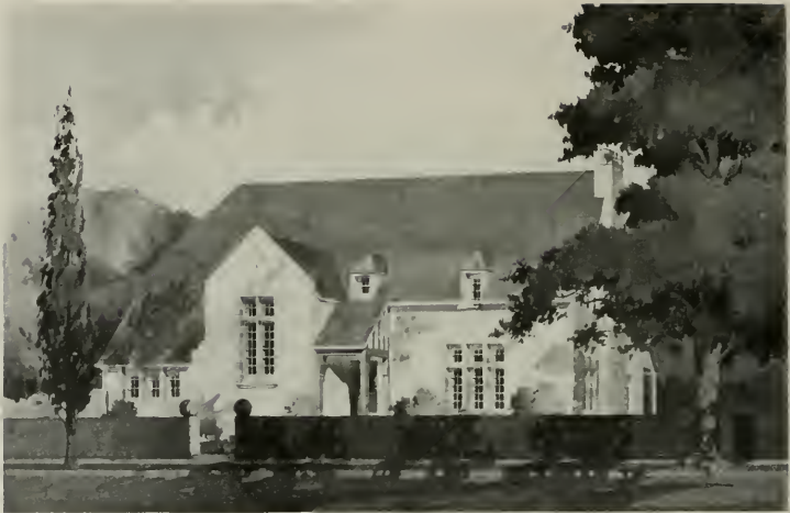
A SOUTHERN CALIFORNIA RESIDENCE Pierpont & Walter S. Davis, Architects
