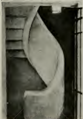
Spiral concrete staircase.
