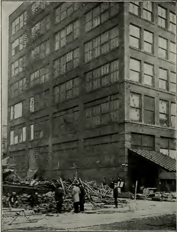
A Successful Fire Stop.—Showing satisfactory fire retardant service of wired glass in metal window frames. Warehouse across twenty-foot alley was totally destroyed. Windows toward rear shown boarded up were broken when side wall of burning building fell.
