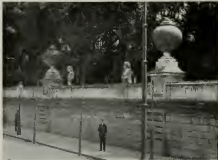
RETAINING WALL, GARDEN OF THE DOWAGER QUEEN'S PALACE, ROME, ITALY
