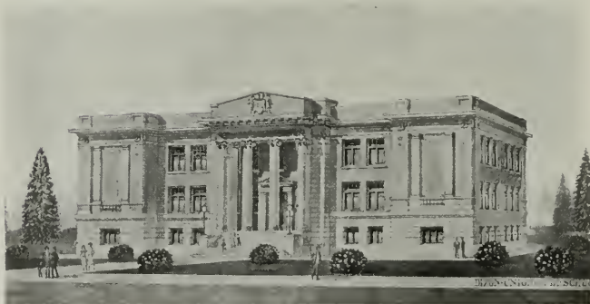
UNION HIGH SCHOOL, DIXON, CALIFORNIA Henry C. Smith, Architect
