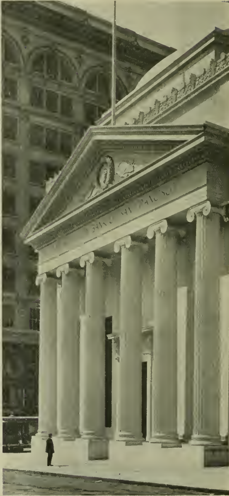
COLONNADE, SAVINGS UNION BANK OF SAN FRANCISCO BLISS & FA'VILLE, ARCHITECTS
