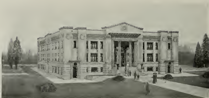
ALTERNATIVE SKETCH, RIO VISTA JOINT UNION HIGH SCHOOL Henry C. Smith, Architect
