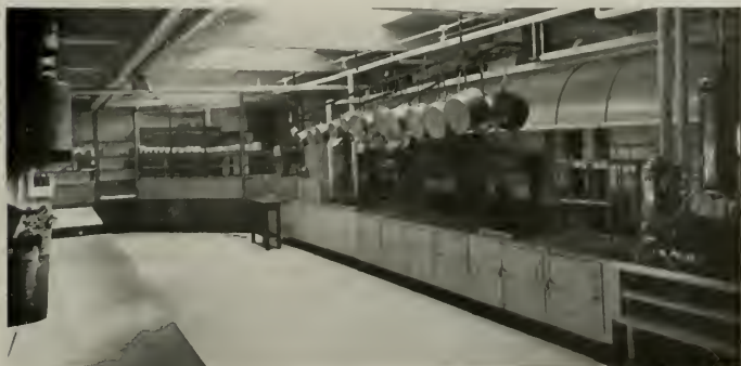
KITCHEN, COMMERCIAL CLUB, SAN FRANCISCO Walter H. Ratcliff, Jr., Architect
