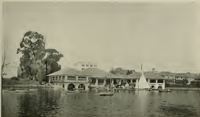
CONCRETE BOAT HOUSE, LAKE MERRITT, OAKLAND Walter D. Reed, Architect
