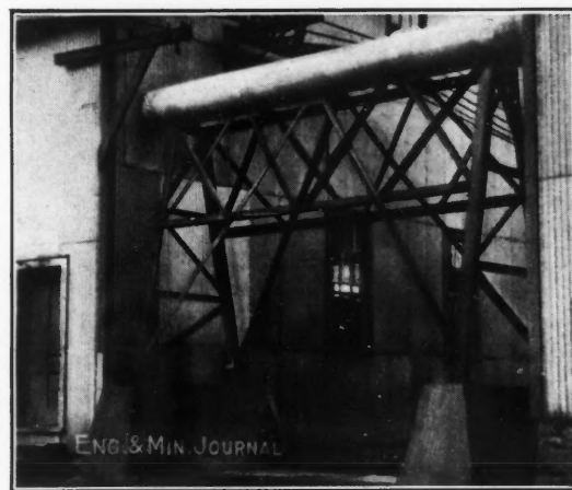
STEEL ANGLE STRUCTURE TO DAMP STEAM-PIPE VIBRATION
