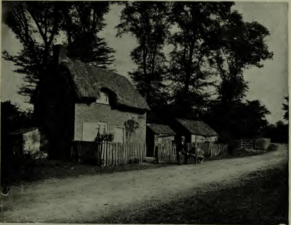
CAR COLSTON GREEN. Commencement of the Green.
