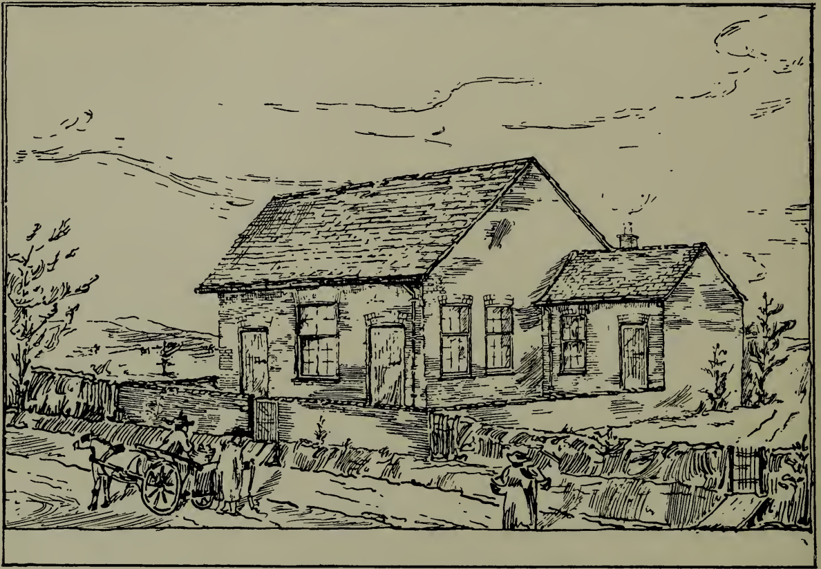
DEAD LANE PRIMITIVE METHODIST CHAPEL, LOUGHBOROUGH. 1818—1837.
