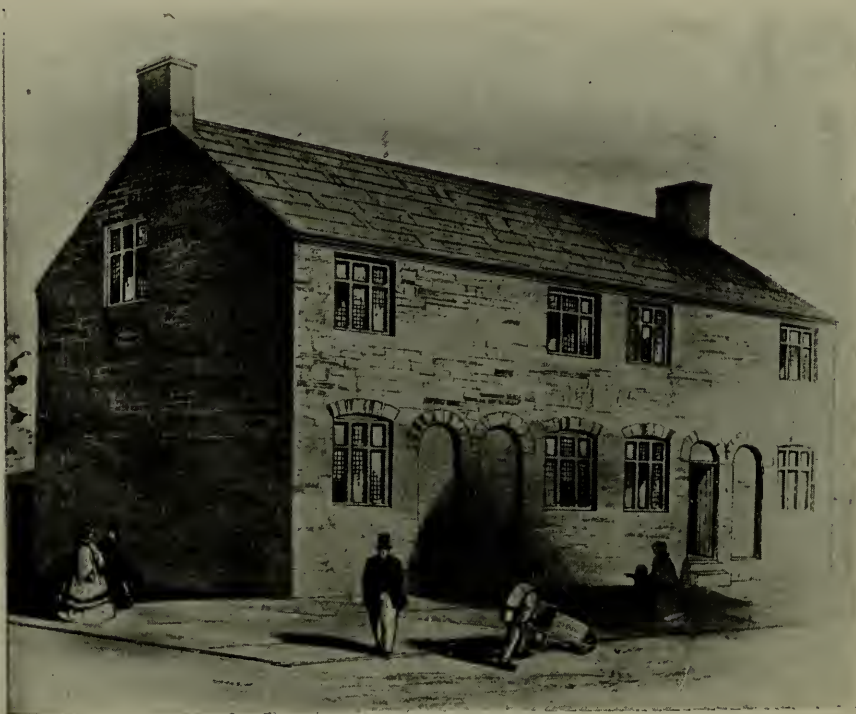
TUNSTALL FIRST CHAPEL.
