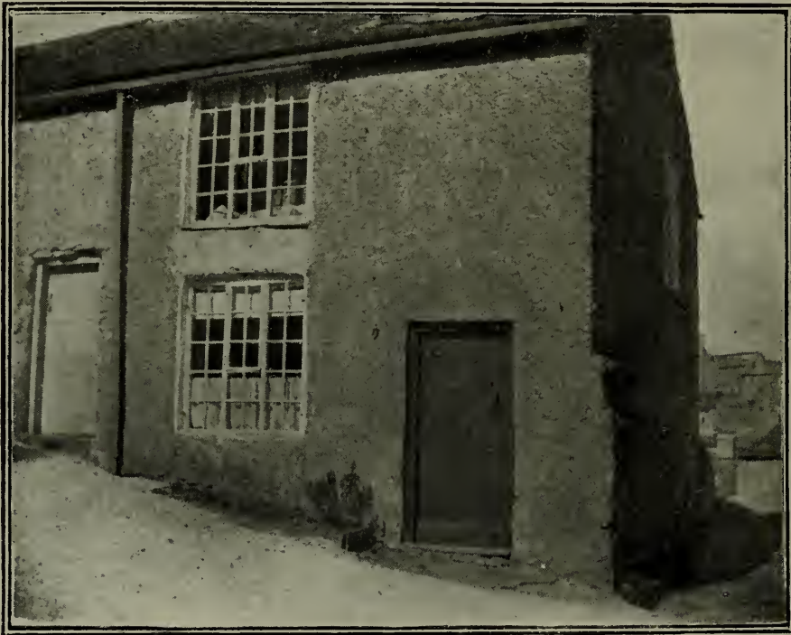
FIRST CHAPEL, BRADWELL.
