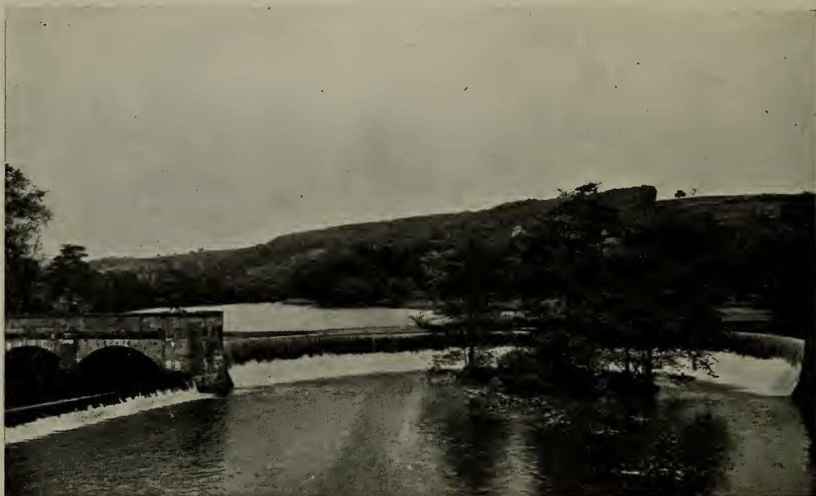
BRIDGE OVER THE DERWENT AT BELPER.
