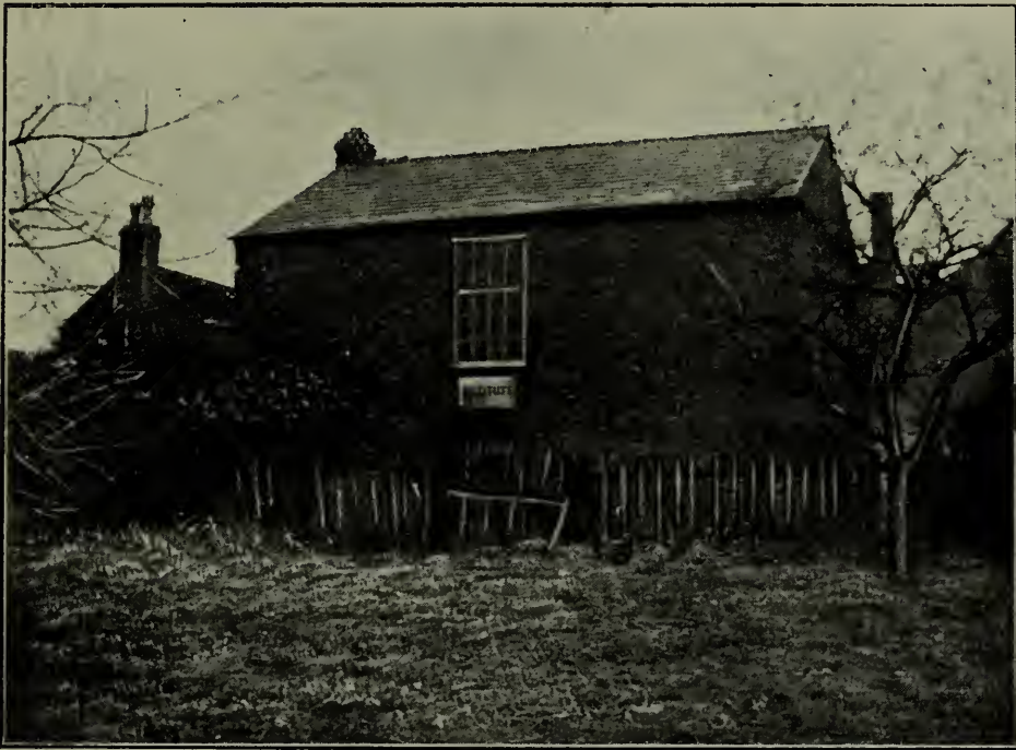
EAST BRIDGFORD OLD CHAPEL.—NOW PUBLIC READING ROOM.
