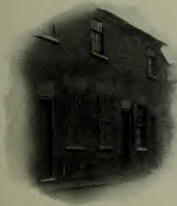
ILKESTON FIRST CHAPEL—NOW TWO COTTAGES.
