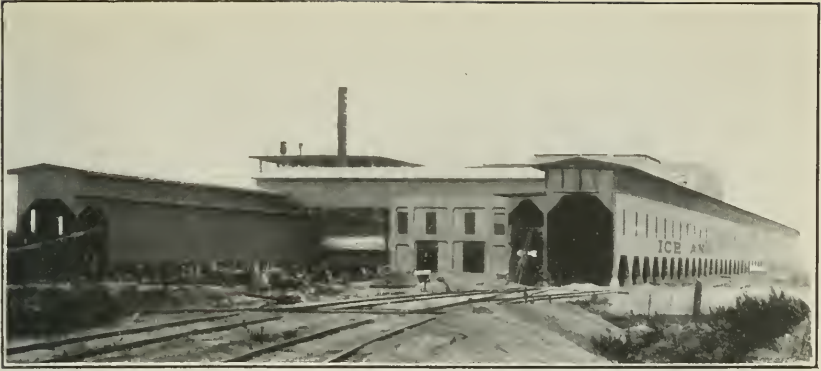
FIG. 1.—GENERAL VIEW OF PLANT FROM THE EAST SIDE, SHOWING PRECOOLING BUILDING AND COVERED AIR DUCTS LEADING FROM IT TO THE CAR SHEDS ON EITHER SIDE.
