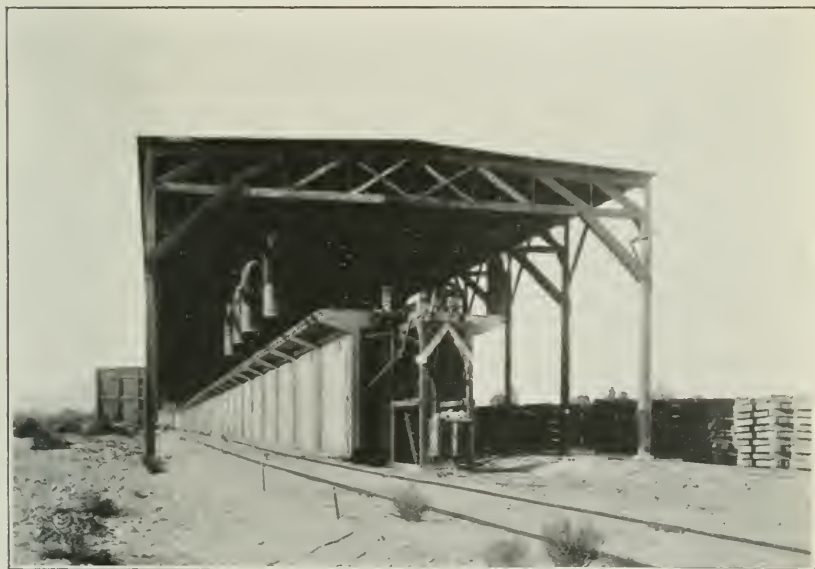
FIG. 2.—END VIEW OF PRECOOLING SHED.
