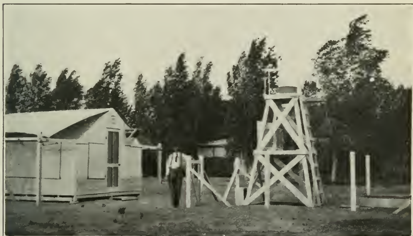
FIG. 3.—OBSERVING STAND, 10 FEET HIGH, FOR STUDYING THE FACTS OF EVAPORATION IN THE UNITED STATES.
