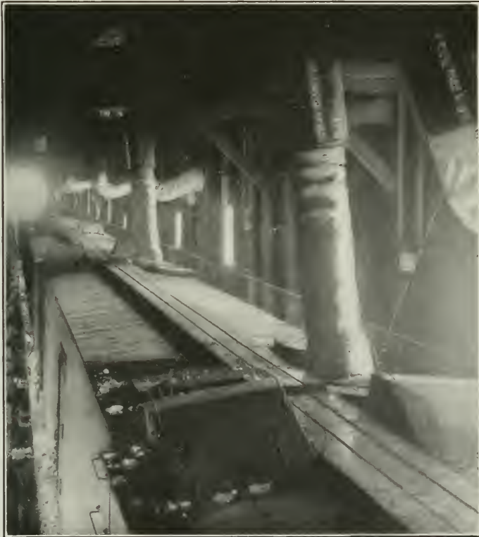
FIG. 2.—INTERIOR OF PRECOOLING SHED, SHOWING FLEXIBLE AIR-PIPE CONNECTIONS FOR WITHDRAWING AIR FROM CARS.
