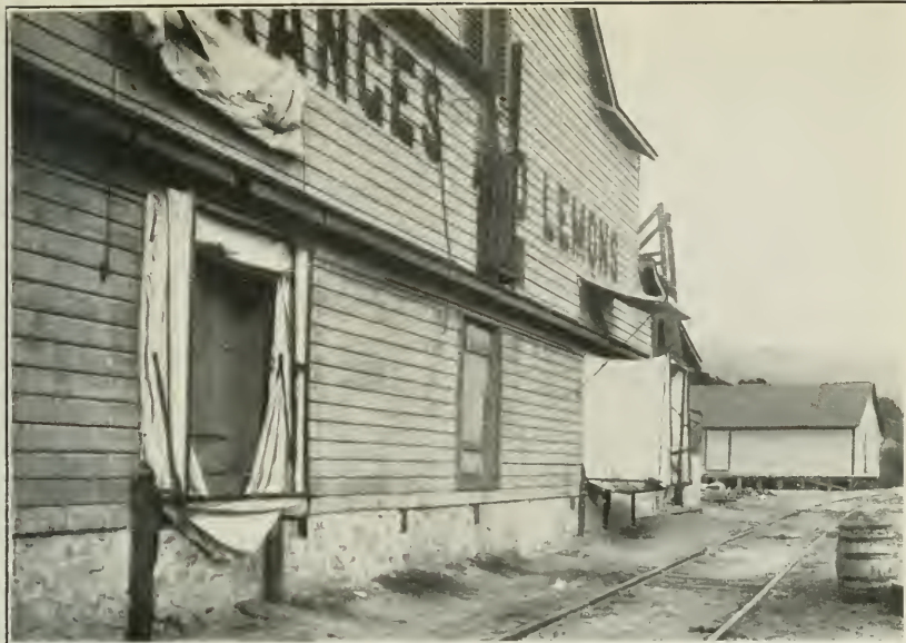
FIG. 1.—CANVAS HOODS USED AT AN ORANGE-PRECOOLING PLANT AT EAST HIGHLANDS, CAL., TO PREVENT LOSS OF COLD AIR IN LOADING PRECOOLED FRUIT INTO CARS.
