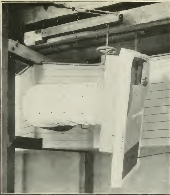
FIG. 1.—ADJUSTABLE DOOR CONNECTION FOR BLOWING COLD AIR INTO DOORWAYS OF CARS, SHOWING CURVED Baffle PLATES FOR DISTRIBUTING AIR INTO UPPER PARTS OF CARS.
