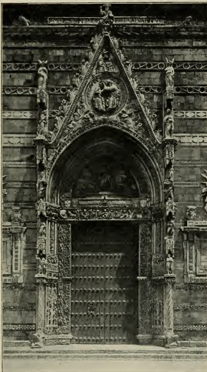
Fig. 386. Messina. Central Doorway of Cathedral.
