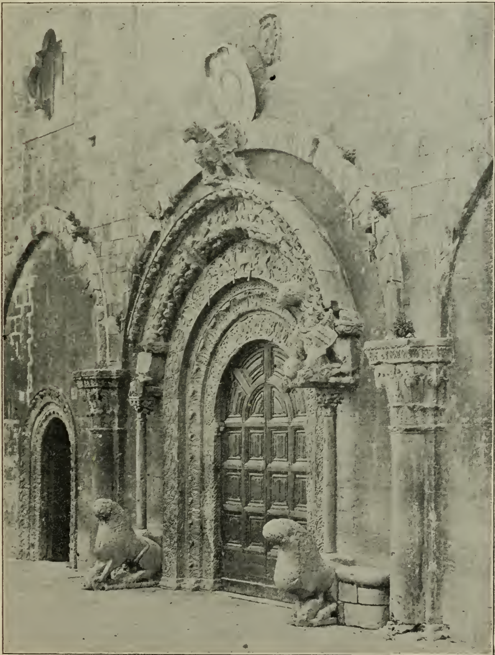
Fig. 277. Ruvo. Central Doorway.
