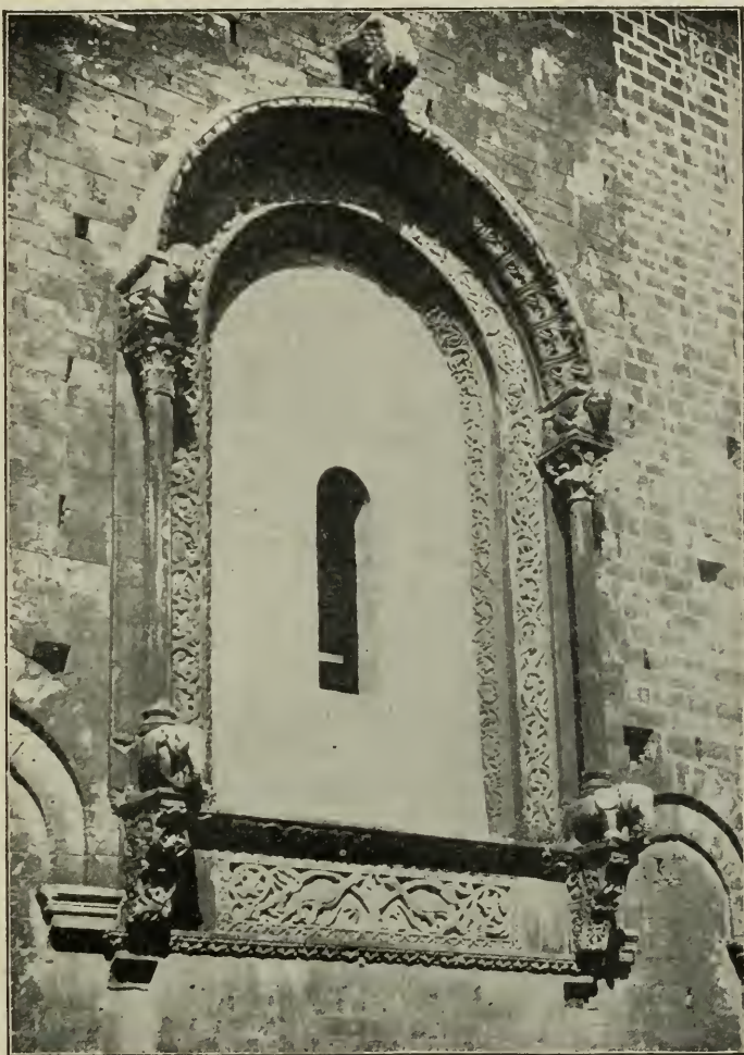
Fig. 278. Bari. Apse Window in Cathedral.
