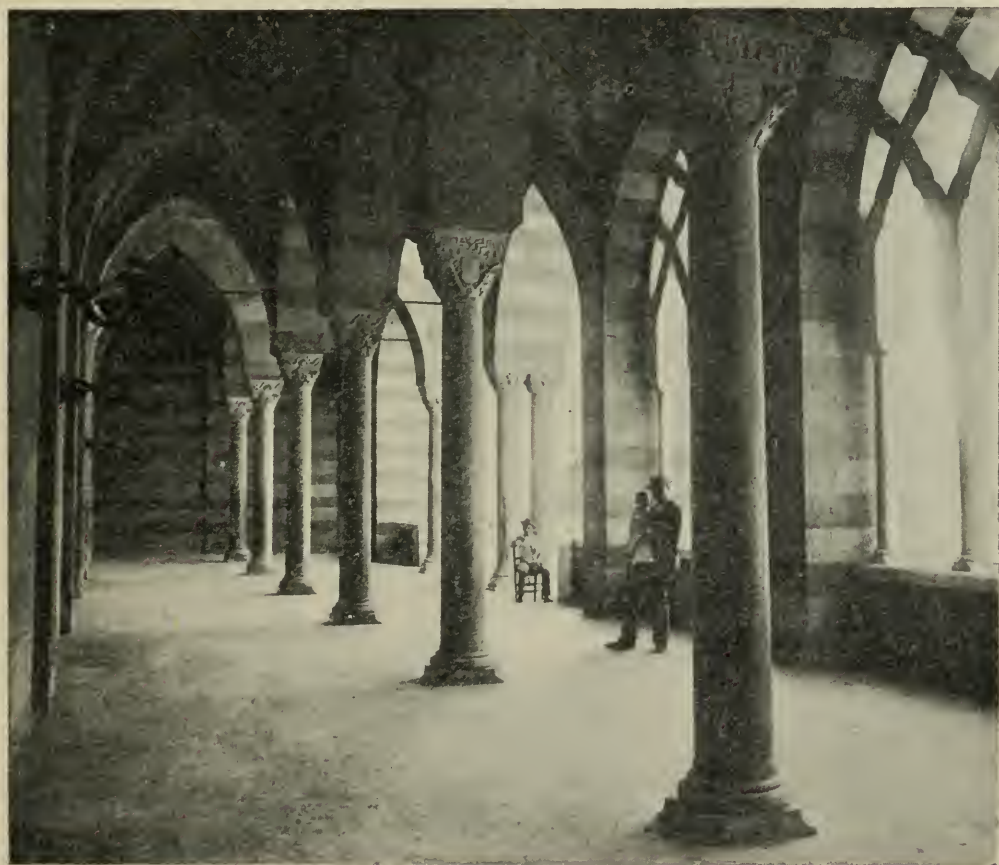
Fig. 269. Amalfi. Interior of Porch.
