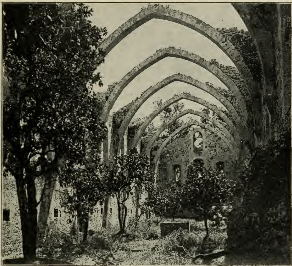
Fig. 333. Fossanova. Interior of Infirmary.
