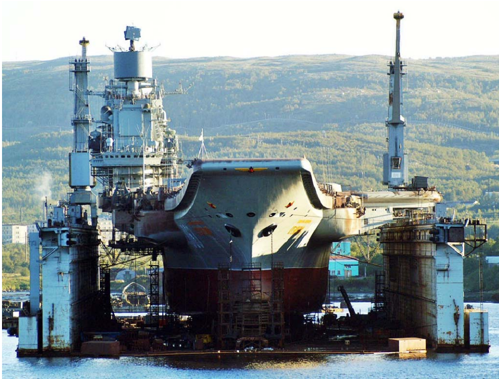
Figure 20. Admiral Kuznetsov inside the PD-50 floating drydock (From Pieter Inpyn, 2010)
