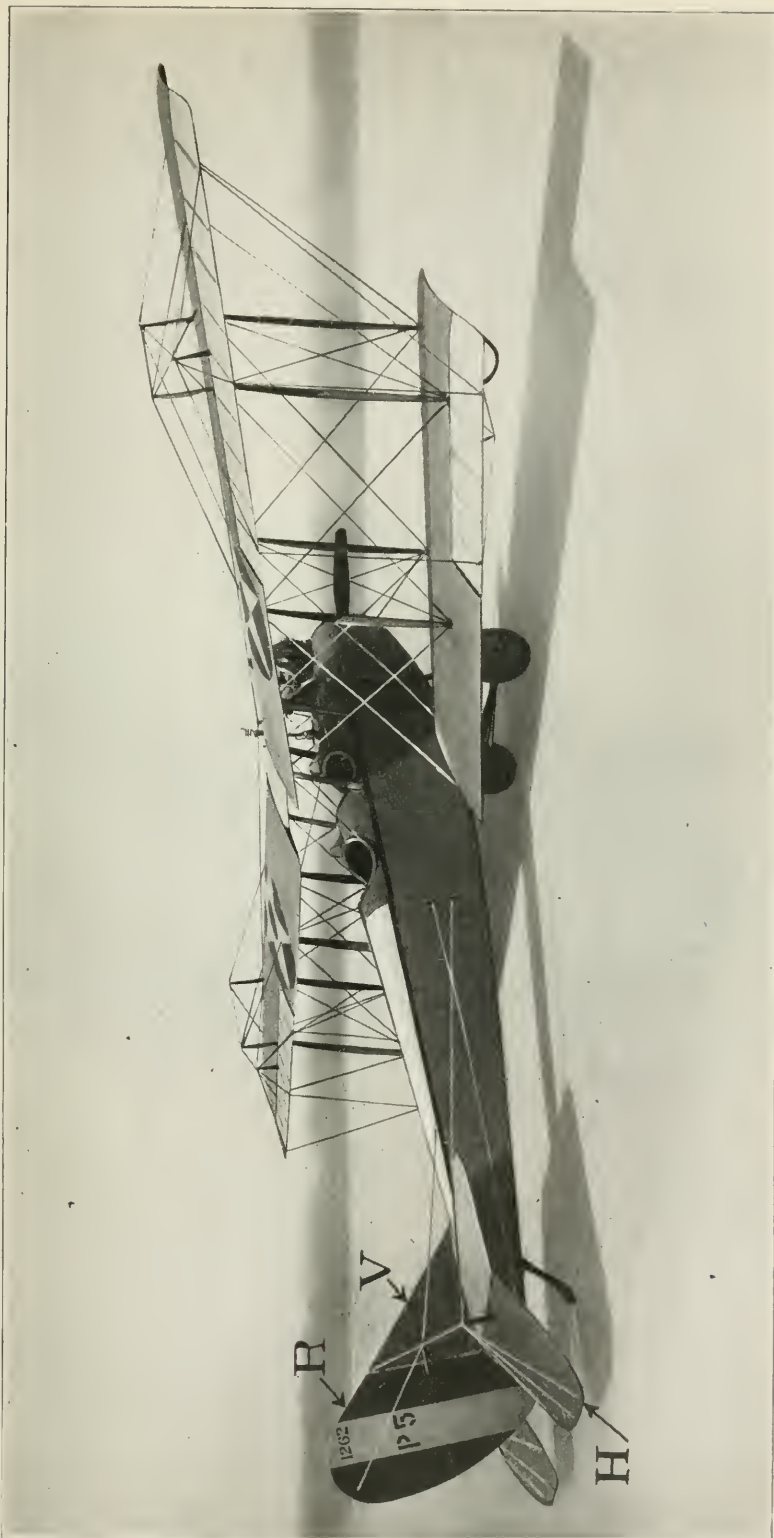
Fig. 6—Curtiss airplane, showing control surfaces
