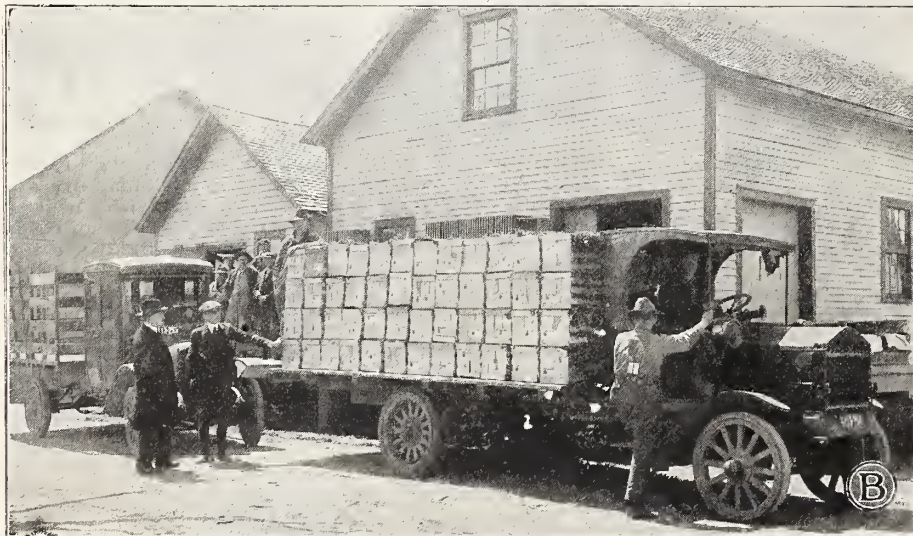
Present Packing Houses, 1923—Baldwin's New Ground Plants Ready for Shipment.
