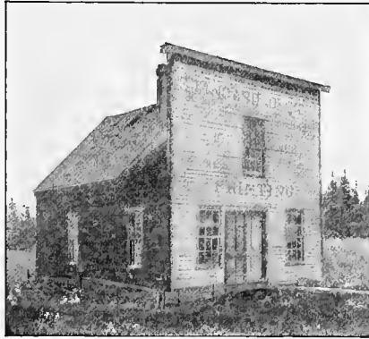
"The first frame structure"
