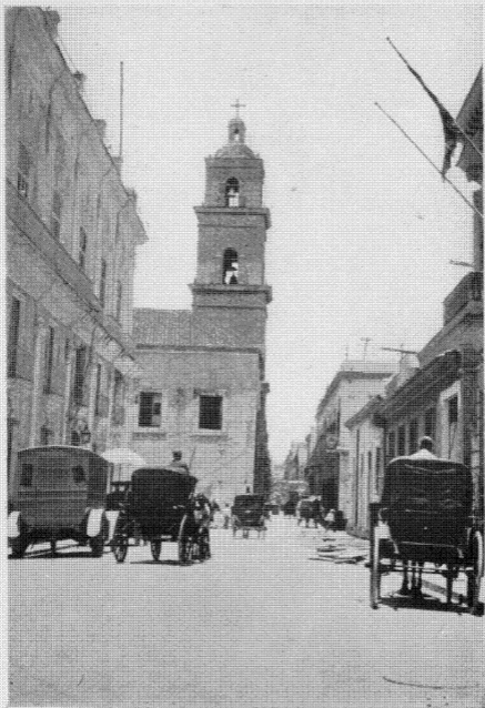
SANTA DOMINGO CHURCH AND O'REILLY STREET, HAVANA
