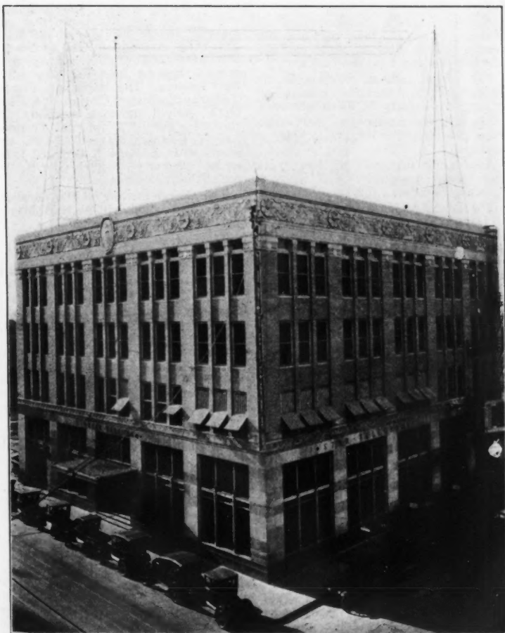
The Star-Telegram building showing the radio antenna. At the end of the installation this antenna, which is only ninety feet in length, was considered entirely too short for nation-wide use. However it was given a test and has proven entirely satisfactory. It is one of the shortest of all antennas used by high power stations and demonstrates that radio transmitters are more nearly perfect than engineers have anticipated.
