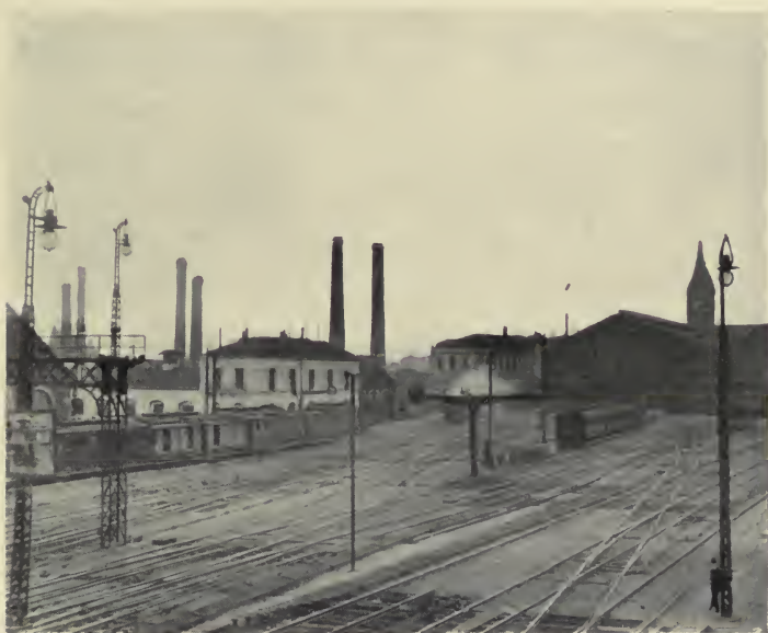
OUTSIDE THE GARE DE LYON.
