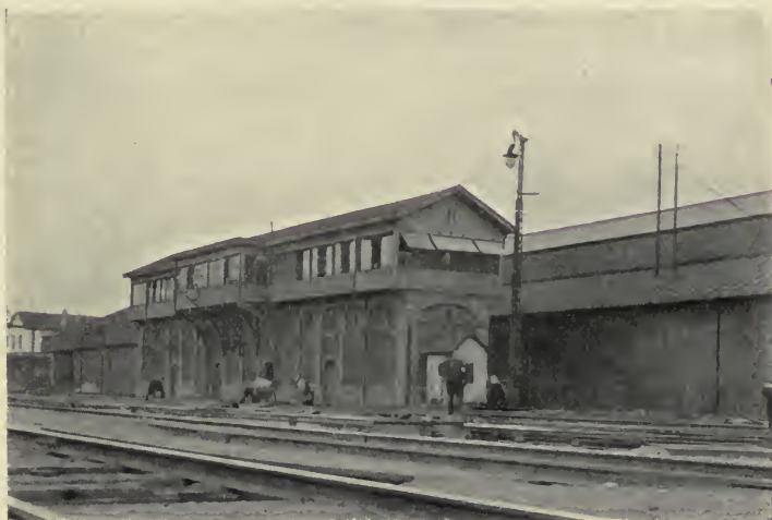
SIGNAL BOX AT THE GARE DE LYON.
