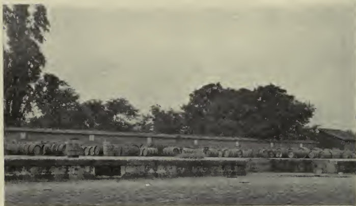
WINE PLATFORM AT P.L.M. GOODS STATION.
