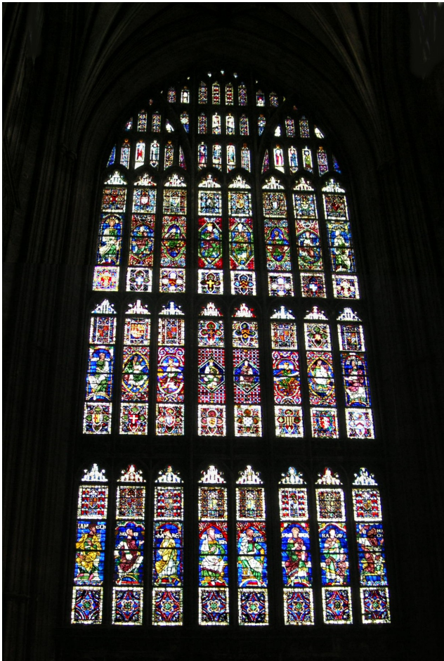
Figure 157 A large Perpendicular style a Gothic b window of eight lights in Canterbury Cathedral c , c. 1400, which contains medieval glass.
