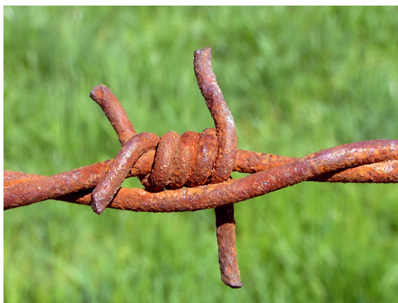
Figure 134 This iron wire has taken years to become rusty.
