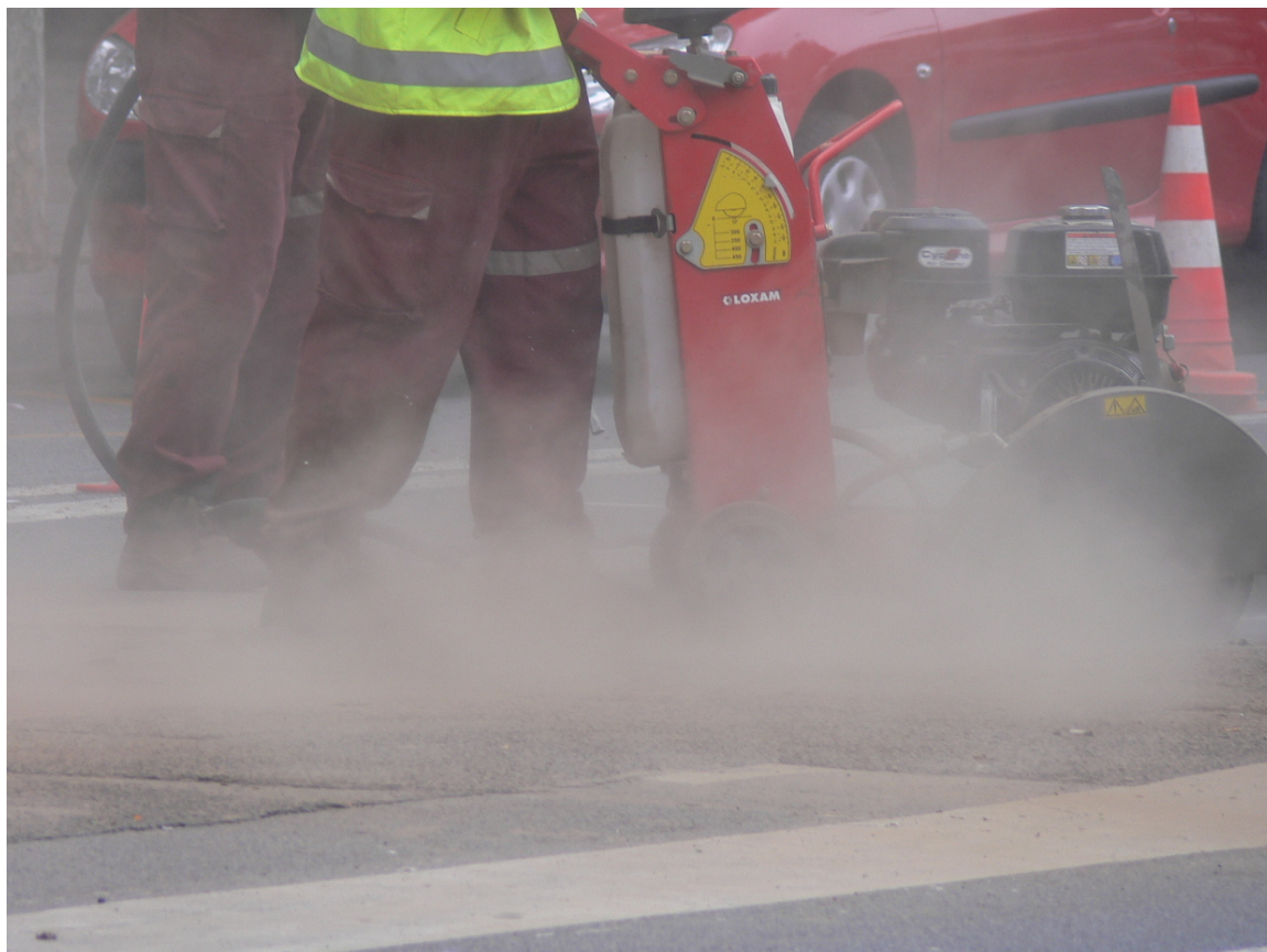
Figure 11 This dust is a suspension because it settles after the work is done.
