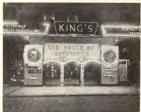
Electrical Front from Shanghai
