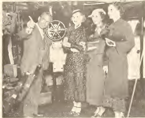
Explorer Starts Loew Cooling Plant
