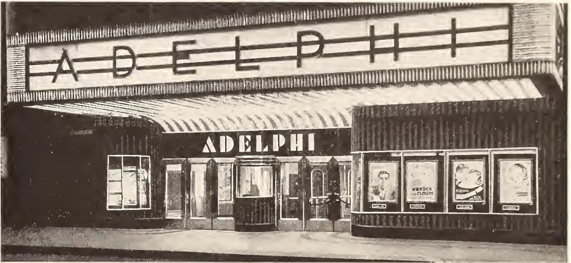
AFTER: And this is the difference a new Pittco Theatre Front made! Architect Mark D. Kulischer, who designed the front, and the theatre manager both feel that "the flash and richness of Pittco materials make them ideal for use on theatre fronts . . . and that the results obtained amply justify the expenditure".
