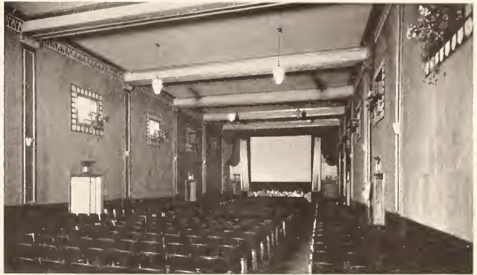
Auditorium of the Regun theatre in New York City, with a decorative scheme incorporating Atlantic Gypsum "Acoustex." The tiles are applied to the side walls and rear wall—there is no acoustical treatment at ceiling. Pilasters, friezes and beams are in ornamental plaster, and the color scheme consists in bronze, gold, silver and green.
