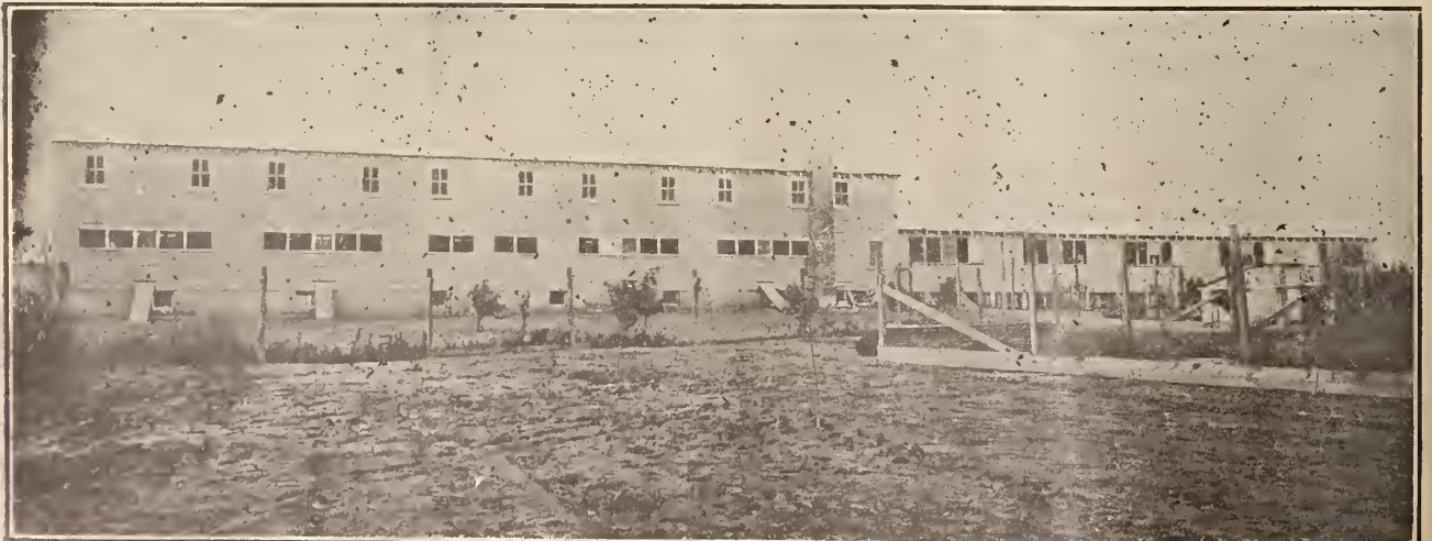
One of the Newtown Producing Company's new laying houses, 212 feet long, divided into two sections, each 100 feet long, with feed house between. Accommodates 1400 birds. Two story section has incubator cellar underneath and Gingseng drying house overhead.
