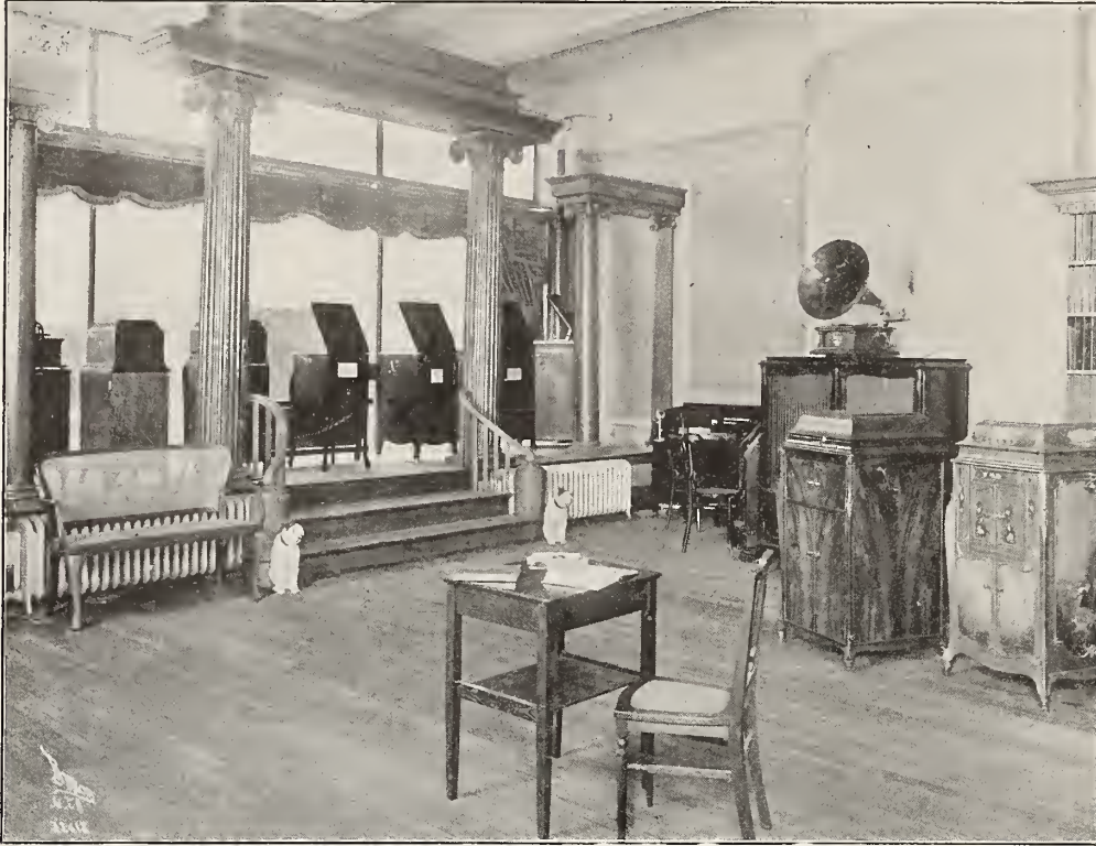
View of Pearsall Warerooms Looking Toward Street.
