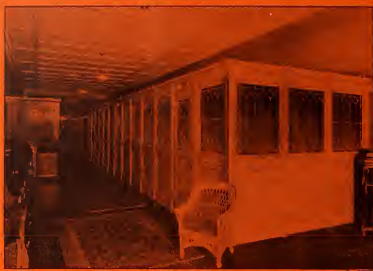
INSTALLATION FOR NEAL, CLARK & NEAL CO.
