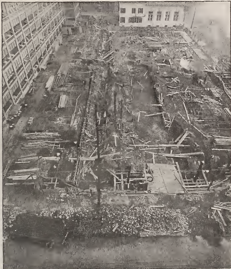
New Shipping Department Under Construction.
