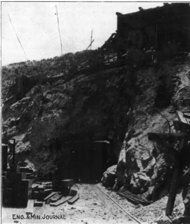
PORTAL OF THE 5000-FT. NIAGARA TUNNEL
