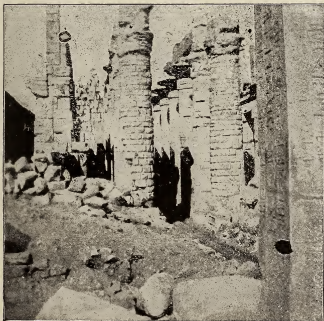
Columns in Temple of Rameses II.
