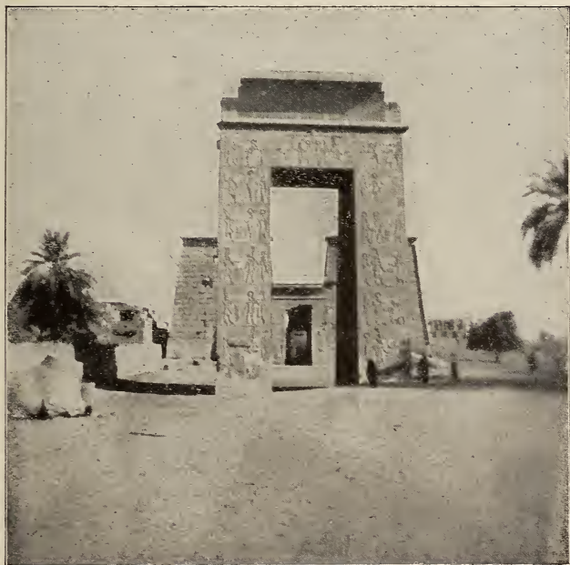
The Pylon of Evergetes I.
