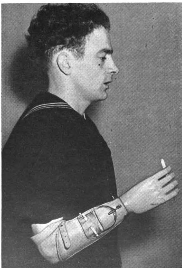
12. Pegs in canals for activating dorsal and volar motors of cineplastic arm.
