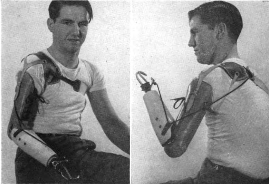
14. Pull on lanyard by opposite shoulder operates utility hook.
