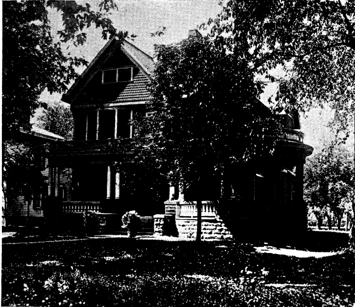
RESIDENCE OF WARREN G. HARDING AT MARION, OHIO
