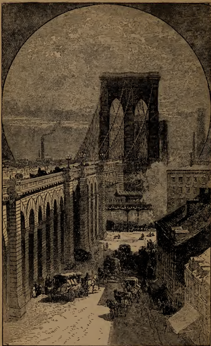
Approach to East River Bridge.
