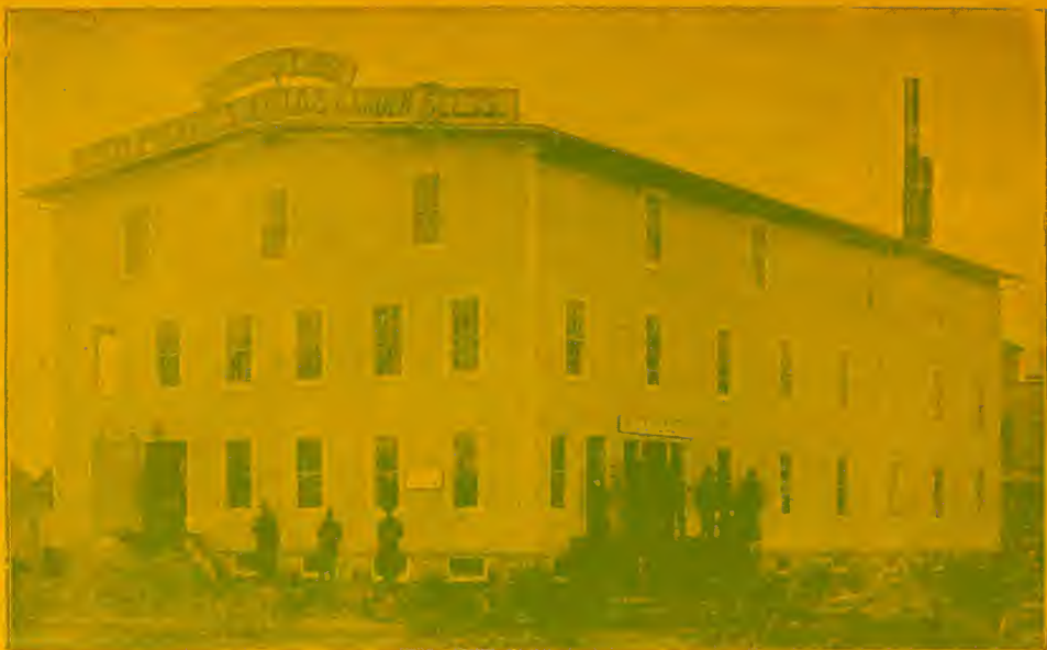
Seed Warehouse at Clinton, on the C. & N. W. Railway.
