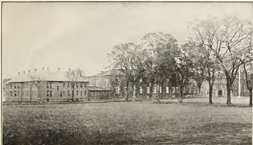
CONNECTICUT STATE PRISON—Situated at Wethersfield.
