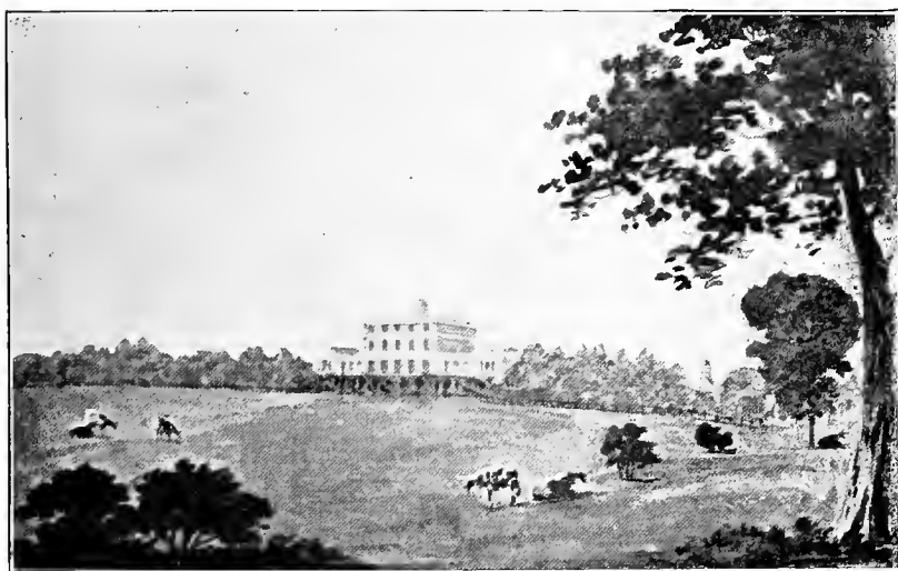
WOODFORD. NO. 2. FROM THE SAME DRAWING BY H. REPTON, SHOWING THE SUGGESTED IMPROVEMENTS.
