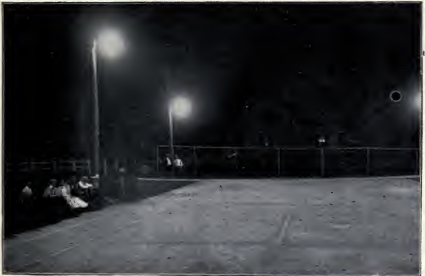
Figure 22—Distribution of light from a D. C. 6.6 ampere enclosed lamp.
