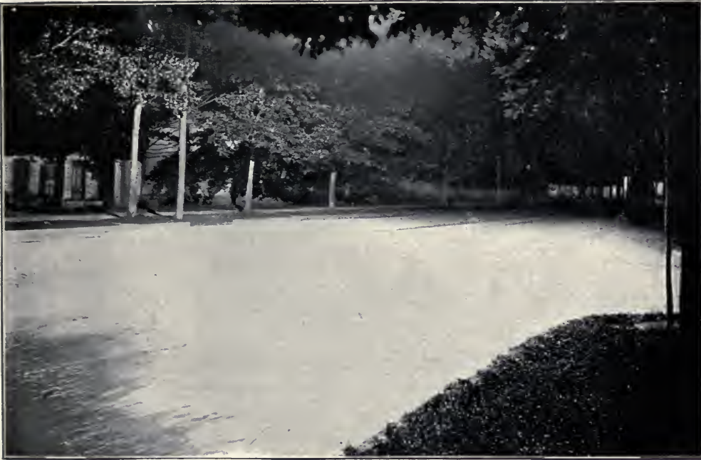
Figure 21—Distribution of light from an A. C. 6.6 ampere enclosed lamp.
