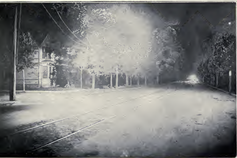
Figure 24—A. C. 6.6 ampere lamps 400 ft. apart.
