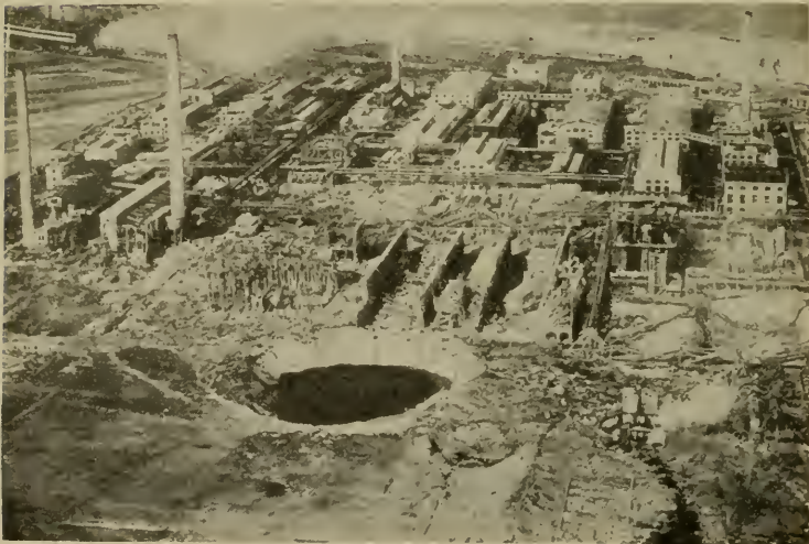
AIRPLANE VIEW OF THE HABER SYNTHETIC AMMONIA PLANT AT OPPAU, GERMANY, AFTER THE EXPLOSION IN 1921
