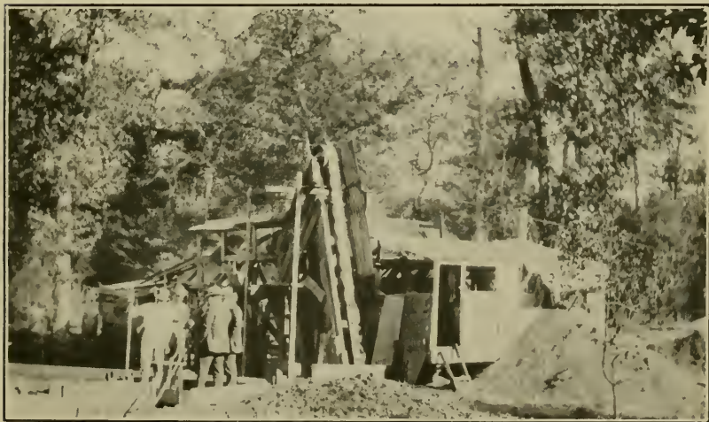
2. DIAMOND PLANT AT THE ARKANSAS MINE
