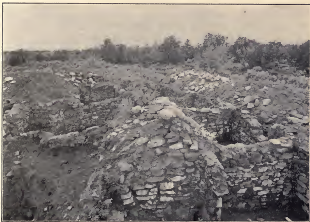
FIGURE 3. — SOUTHEAST END OF NORTH WING.
